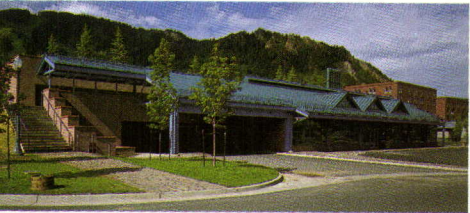
Honor Award Rio Grande Transportation Center Aspen, Colorado RNL Design, Architects
