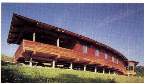
Honor Award Ashland Nature Center Ashland, Delaware Homsey Incorporated, Architects
