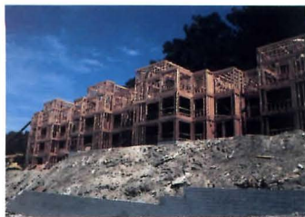
Wood-frame construction delivers cost-effectiveness in high density areas and difficult terrain.
