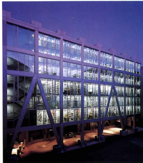
Certificate of Merit MIT Library of Art, Architecture, and Planning Cambridge, Massachusetts Schwartz/Siver Architects
