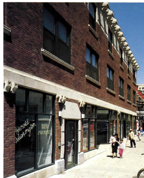
WAYNE CABLE/CABLE PHOTOS
