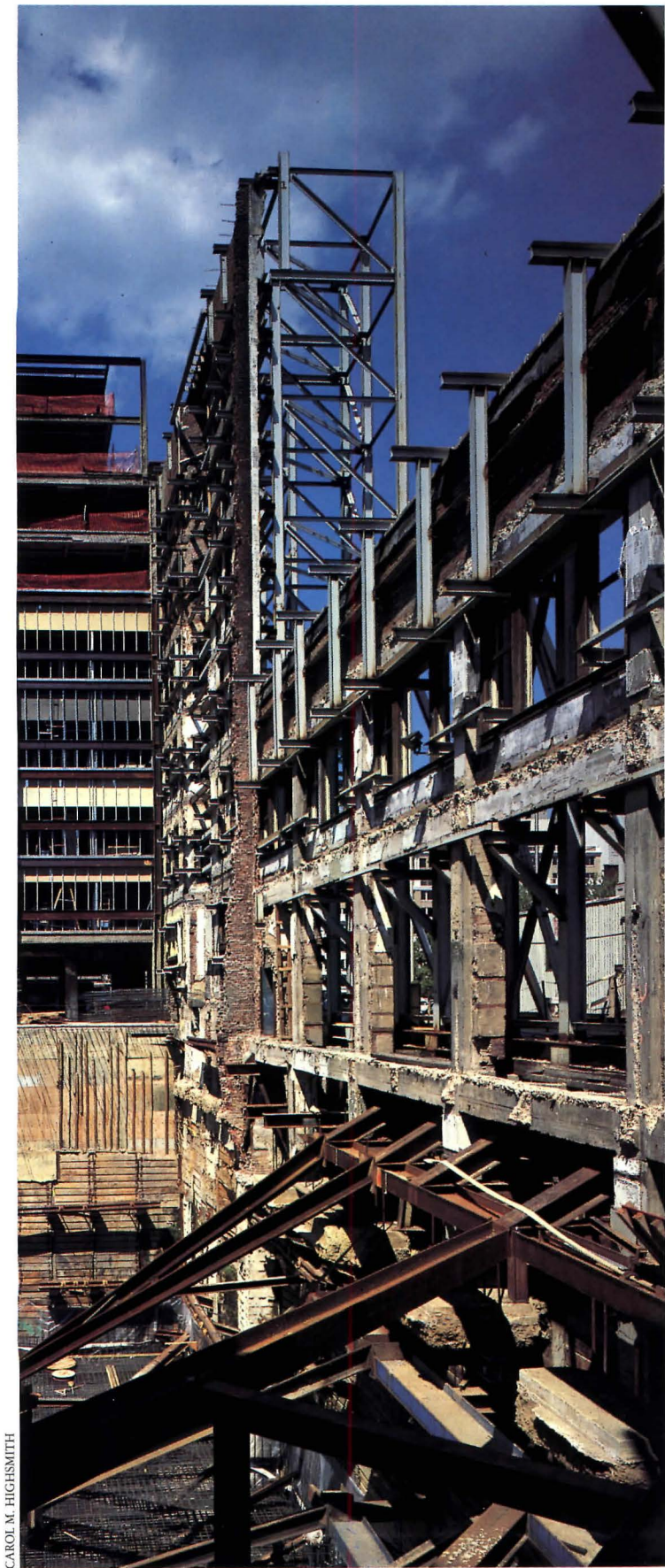
WALL BRACING DETAIL (BUSCH BUILDING)
