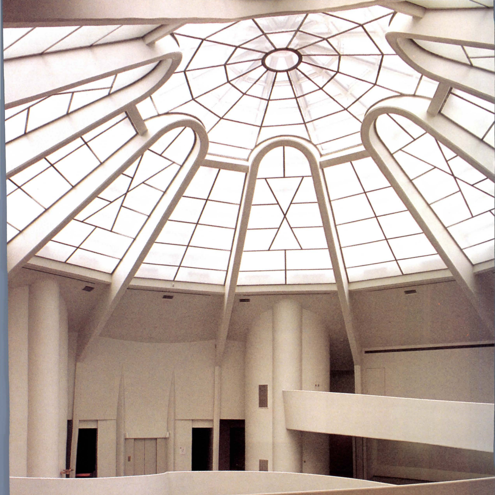
skylight over large rotunda (this page) has been replaced by thermal glass. Light sculpture by artist Dan Flavin (facing page, top left) celebrates Wright's magnificent space. Original V-shaped public stair (facing page, top right) has been refurbished.
