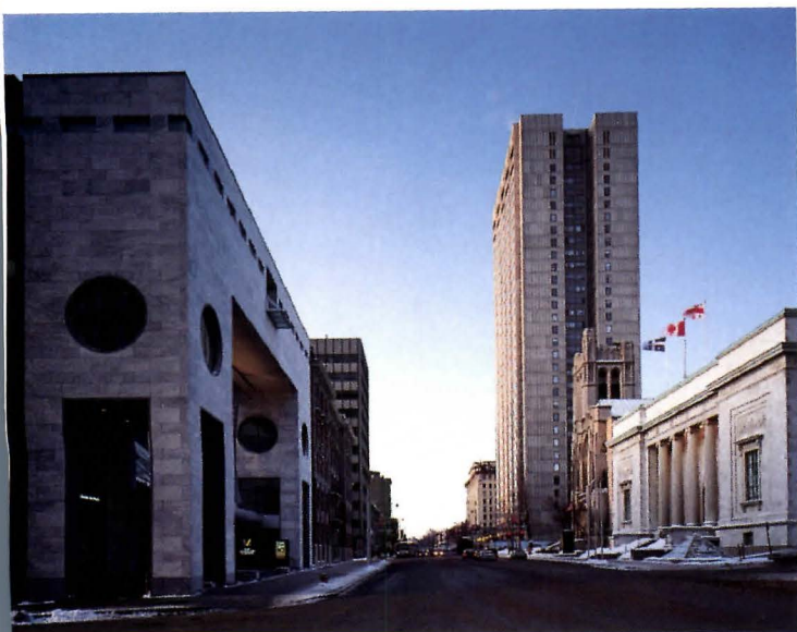
Moshe Safdie's new pavilion (left in photo) for the Museum of Fine Arts connects to the original museum (right in photo) by a tunnel.
