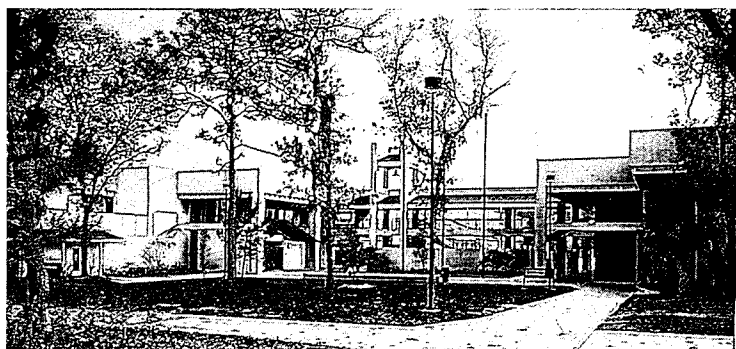
Merit Award, Lay Jury High School West, River Ridge Campus Pasco County, Florida Ranon & Partners, Architects
