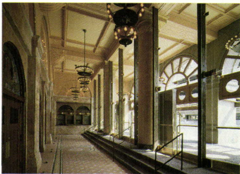
Booth/Hansen reinvigorated Adler & Sullivan's 1888 Auditorium Theatre by inserting fan-shaped steel ornaments and lights into three stone arches at the entrance (top), and adding new chandeliers in the lobby (above).
