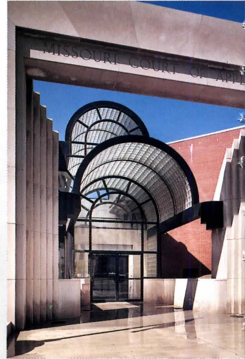
Missouri Court of Appeals, Kansas City, MO Architect: Abend Singleton Associates, Inc. DECORA® Pattern
