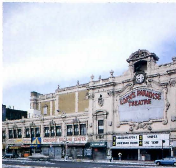
MAIN ENTRANCE: Adjacent to theater.
