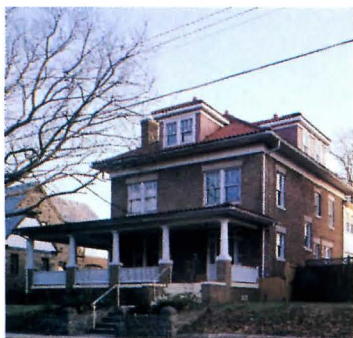
NORTH ELEVATION: Neighboring appearance.
