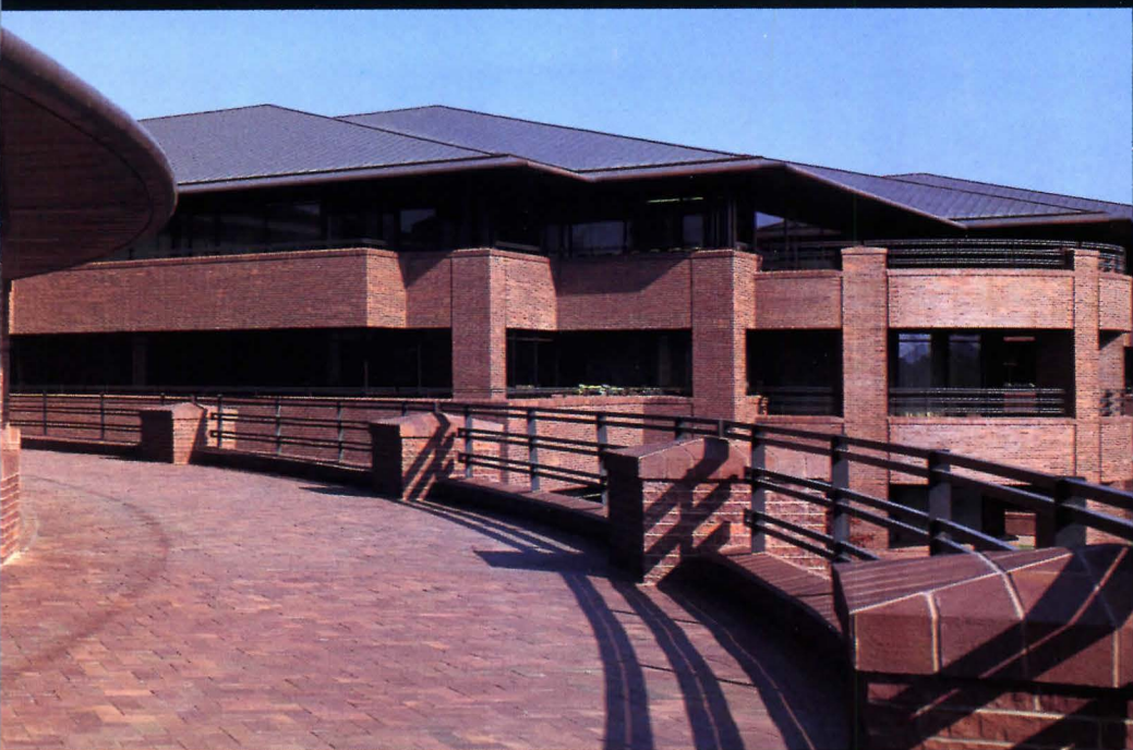
ConAgra Corporate Complex —Omaha, NE Architect: Opus Corporation—Minneapolis, MN
