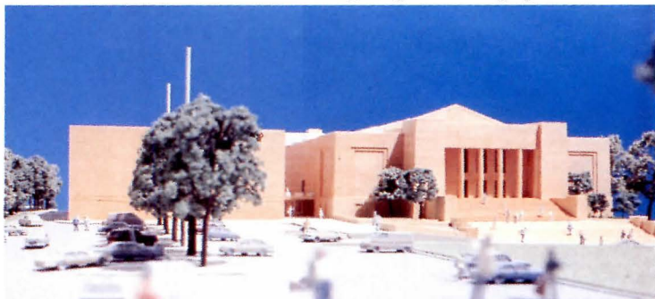
EAST ELEVATION: Addition (left) will be clad in same marble as 1931 structure.
