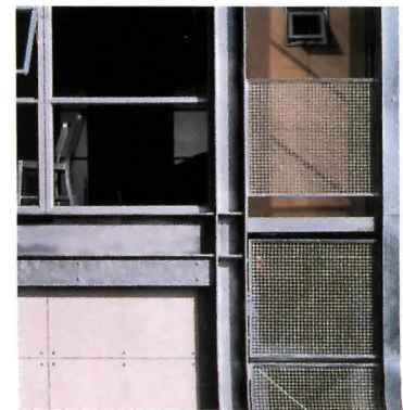
INDUSTRIAL MATERIALS: Exposed steel.
