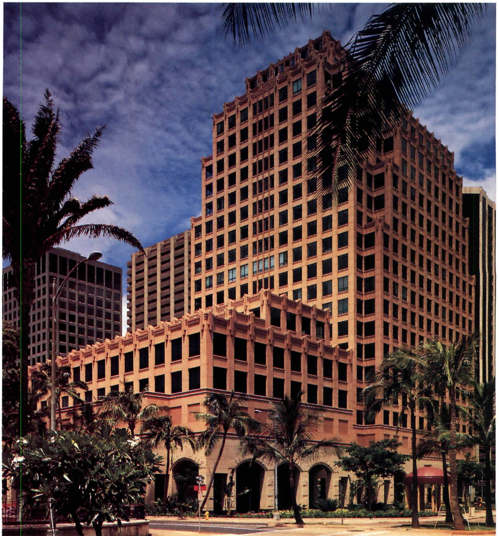
VIEW FROM SOUTHEAST CORNER: Limestone and granite are simulated in precast concrete.
