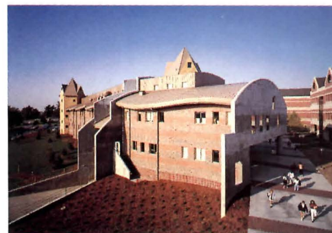
FACING PAGE: Undulating east wall of the Fine Arts Building is composed of brick fabricated in a local beehive kiln. South tower, clad in Minnesota limestone, houses elevator and stairwell.
