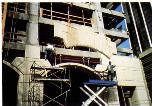
ARCH: Precast panel erected over formwork.
