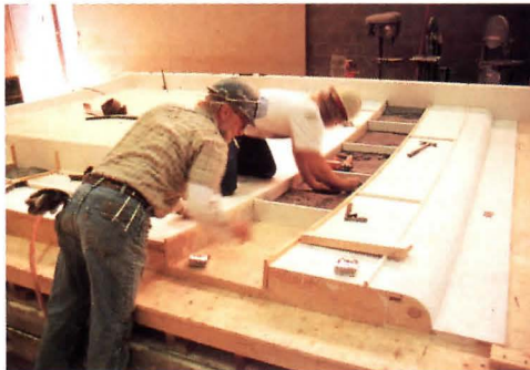
FORMWORK: Urethane forms vary within panel molds.
