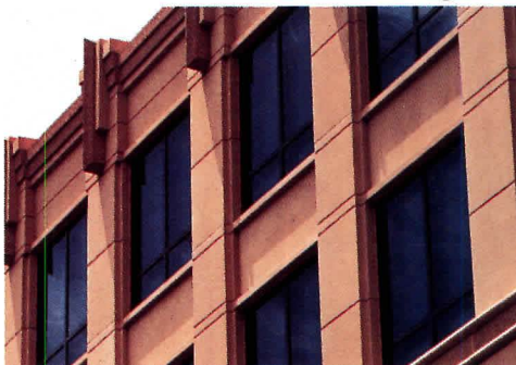
CORNICE DETAIL: Finials cast in fiberglass molds.
