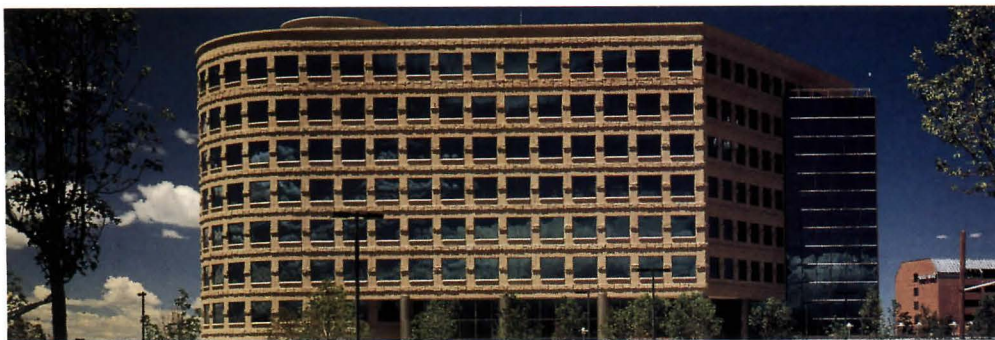
WEST ELEVATION: Travertine marble is replicated in textured precast concrete.
