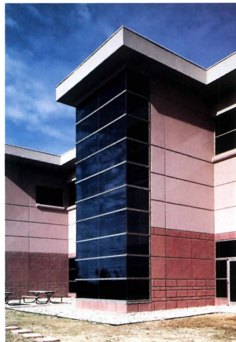
STAIR TOWER: 10-by-30-foot precast panels.
