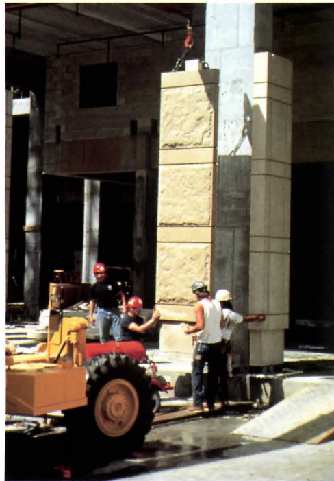
COLUMN: Precast panels enclose concrete structure.
