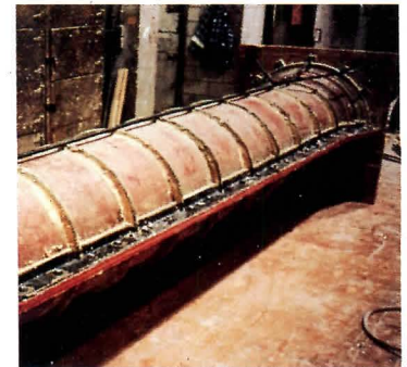
COLUMN MOLD: Formed from fiberglass.
