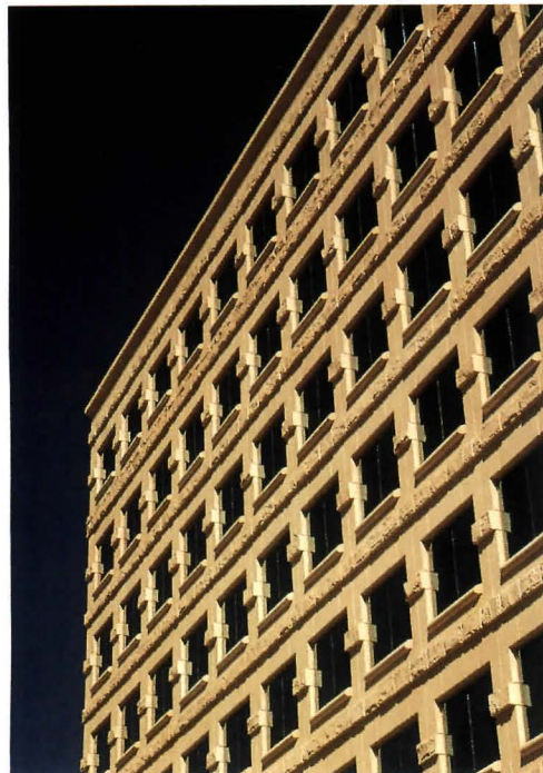
WINDOWS: Bullnose sills are cast within wall panels.
