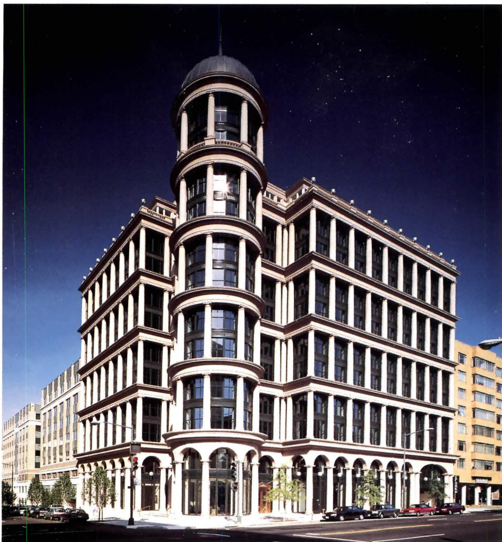
SOUTHEAST CORNER: Precast concrete is designed to emulate Indiana buff limestone and cast iron.
