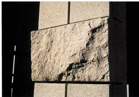
WALL DETAIL: Irregularly cleaved simulated stone.
