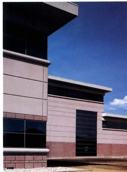
WEST ELEVATION: Bullnose sills visually reduce height.
