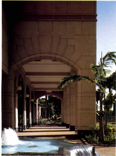
ARCADE: Fiberglass beams create coffered ceiling.
