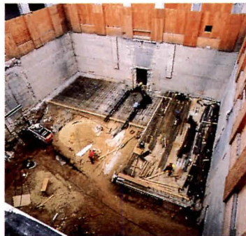
EXCAVATION: New labs and archives.
