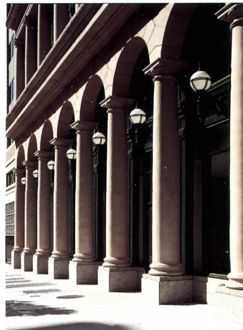
COLUMNS: Each poured as a single piece.
