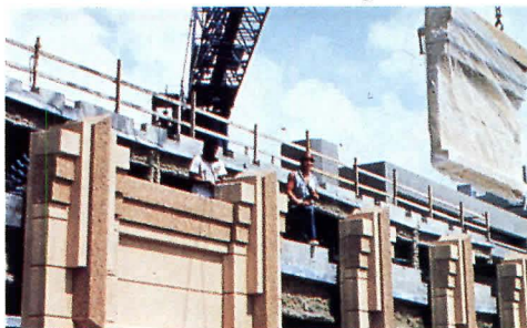
WALL CONSTRUCTION: Panel is lowered into place.
