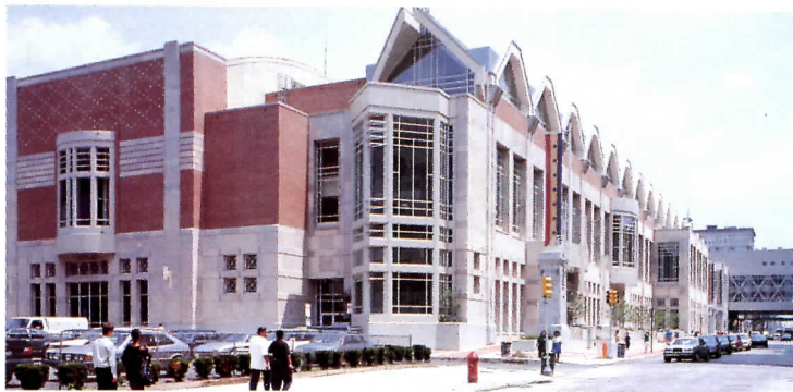
SOUTHWEST CORNER: Bay windows and ridge roofs fit into streetscape.
