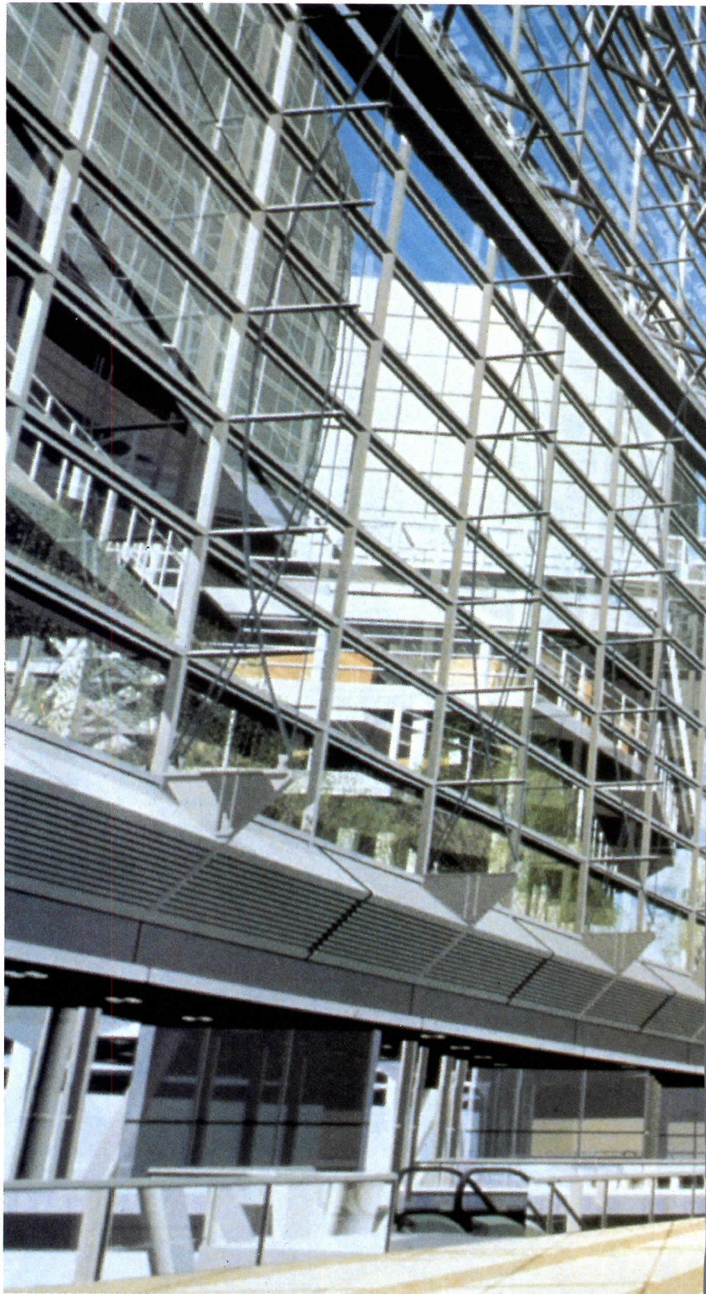
GLASS HALL: Ramps and bridges laterally brace 190-foot-high glass wall supported by cable-tensioned trusses.
