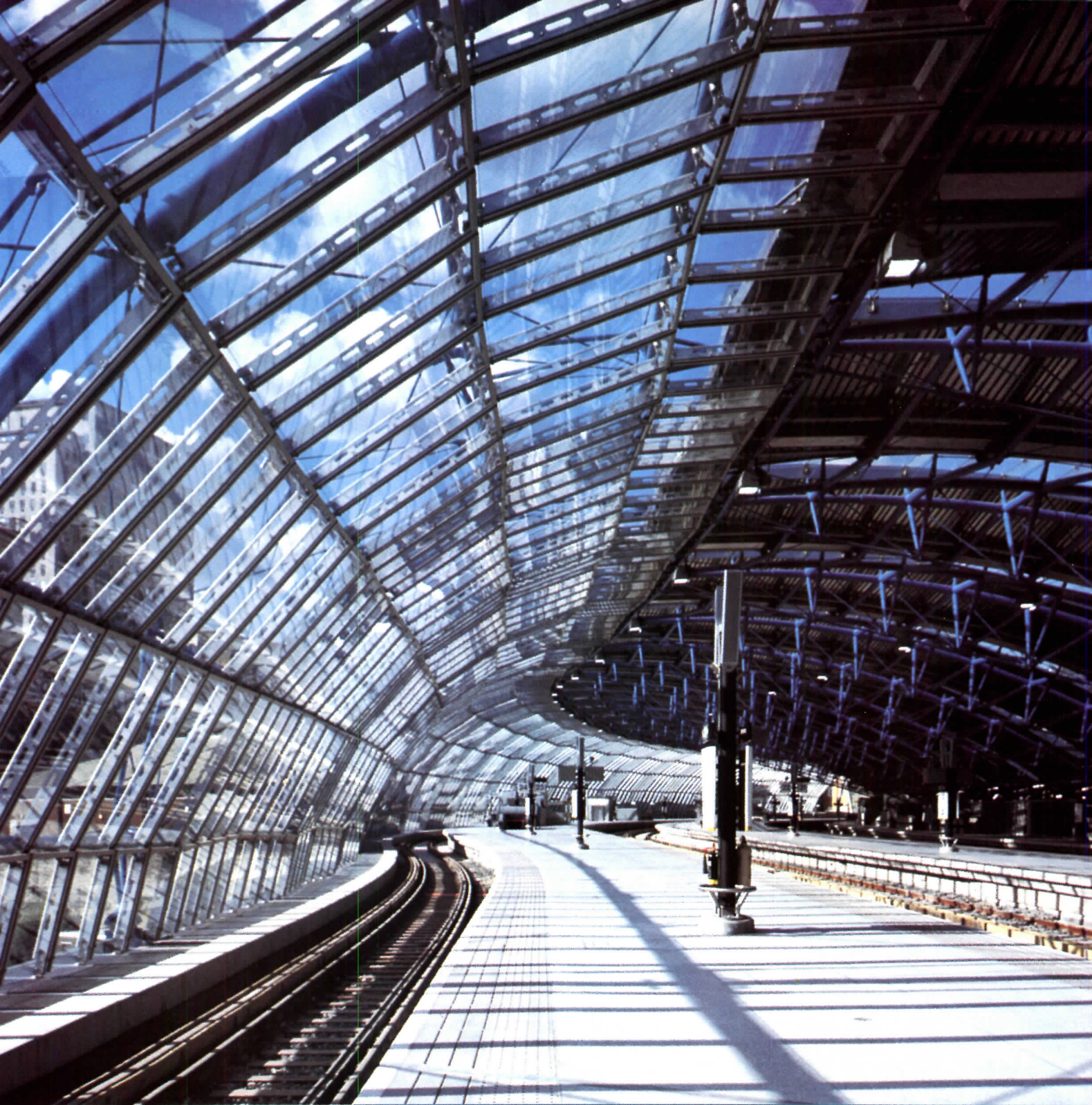
ABOVE: Western half of platform canopy comprises hanging glass panels stiffened with glass fins to eliminate structural mullions and bracing. LEFT: Waterloo International Terminal stretches 400 meters from east to west.
