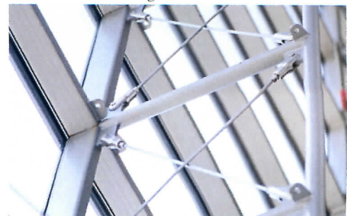
VERTICAL TRUSS: Tensile steel X-bracing.
