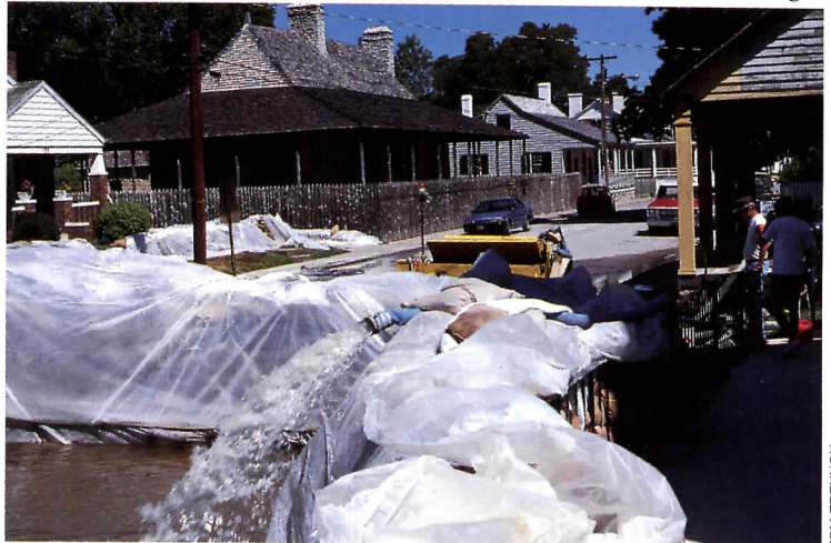
STE. GENEVIEVE: Sandbags helped to save 1770 Bolduc House and its fence.
