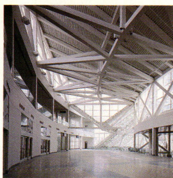
CONCOURSE: Clerestory and trusses.
