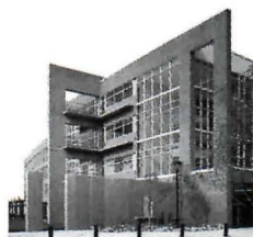
This 325,000 sq ft reinforced concrete building was completed within 17 months.
