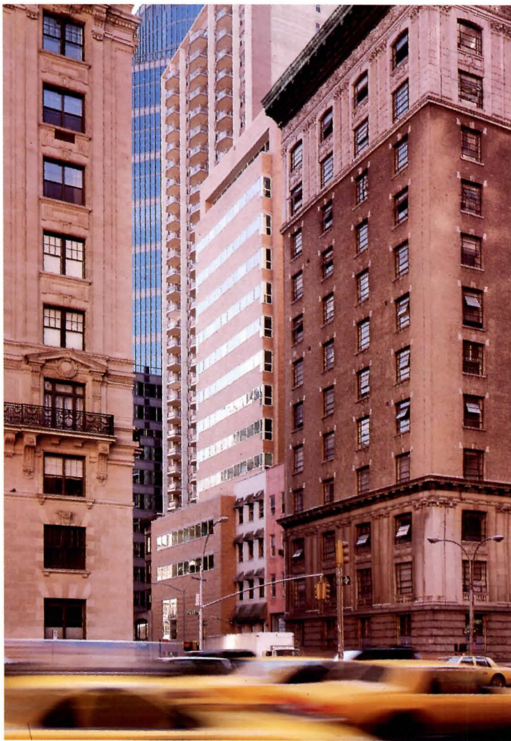
FACING PAGE: The Lighthouse, which spans a mid-Manhattan block, consists of a 1964 structural frame sheathed in a new brick-veneered skin. The redesigned facades have increased window surface, thereby maximizing the level of daylight within. New two-story base fills a former plaza on 59th Street. ABOVE: Base of north facade replaces a demolished six-story building added to the headquarters in 1950.
