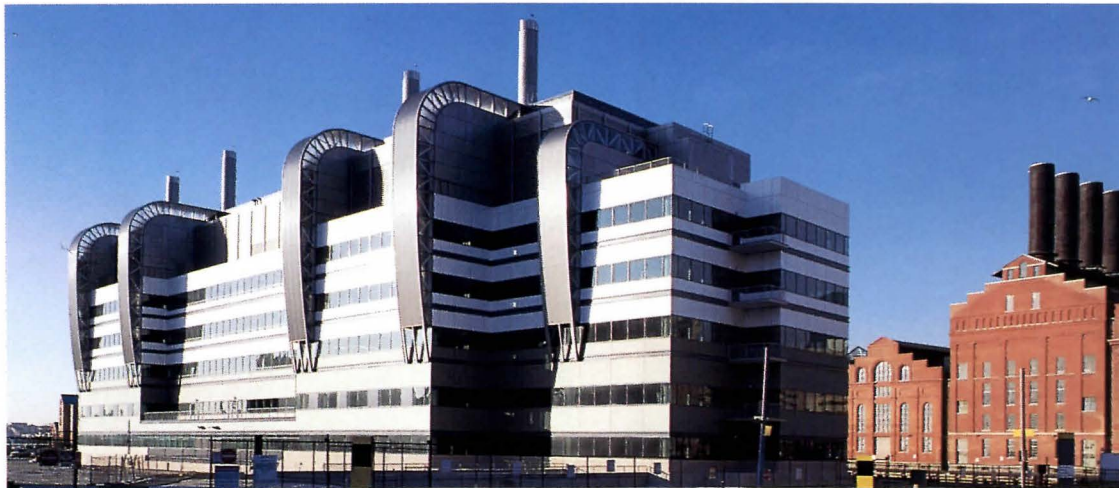
RESEARCH SIDE: Metal-clad block, punctuated by curving hoods for fume exhaust, houses laboratories.
