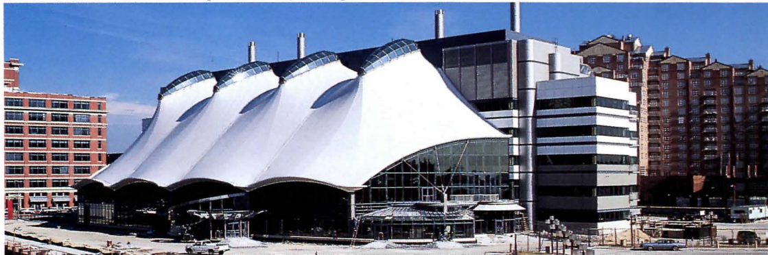
EXHIBIT SIDE: Teflon-coated fiberglass canopy will enclose public Hall of Exploration.
