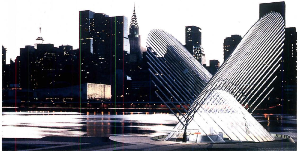
METALLIC WINGS: Computer-operated aluminum fins rotate according to sun's angle to control sunlight in restaurant.
