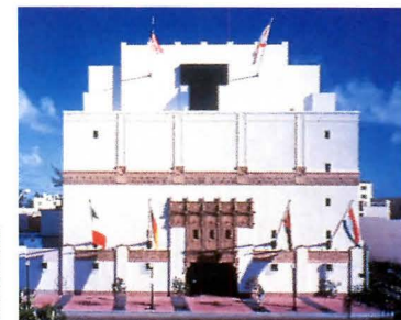
WOLFSONIAN: Former warehouse.
