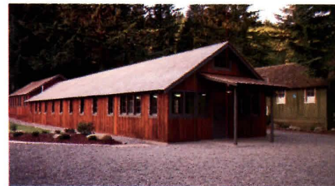
CAMP WASKOWITZ CABIN, MENG ARCHITECTS
