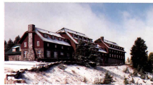
NATIONAL PARK LODGE, FLETCHER FARR AYOTTE ARCHITECTS
