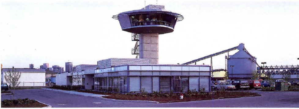
British Columbia Rail Offices and Control Tower North Vancouver, British Columbia Busby Bridger Architects
