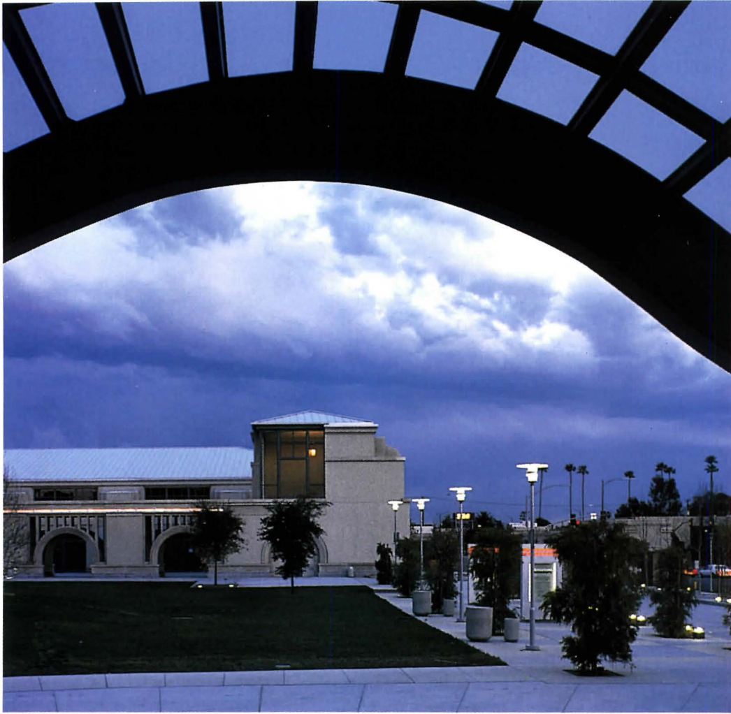
Escondido Civic Center, Escondido, CA. Architect: Moore Ruble Yudell, Architects & Planners, Santa Monica, CA.
