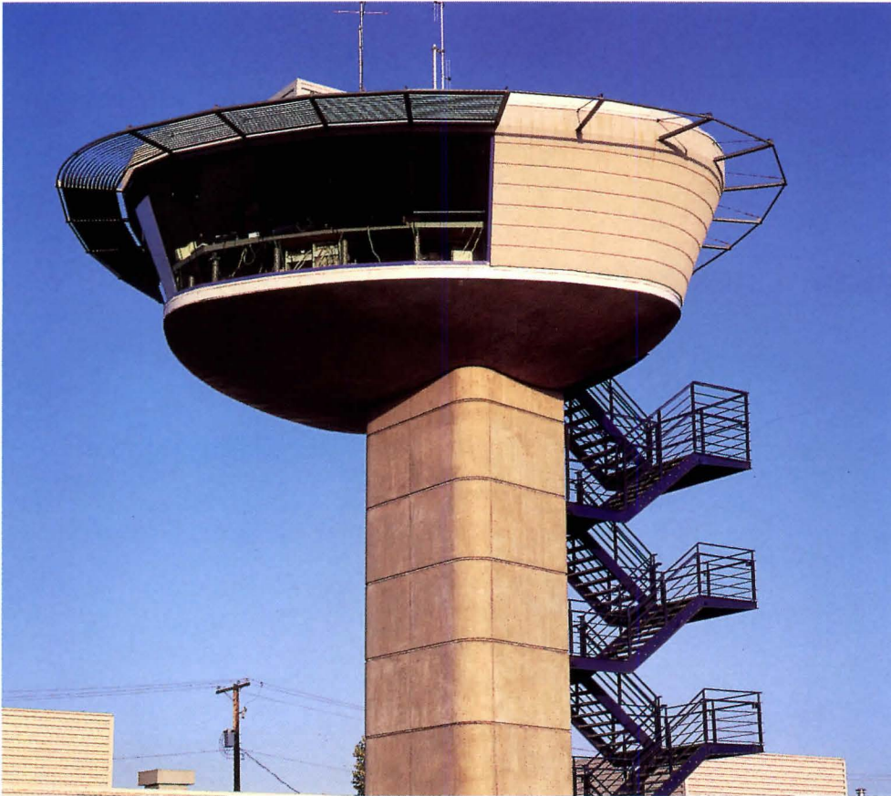
TOP: One-story office building is marked by modular facade. ABOVE: Double curve of control-room slab and steel cornice distinguish tower. SECTION: Functions are hierarchically divided into office block and tower.
