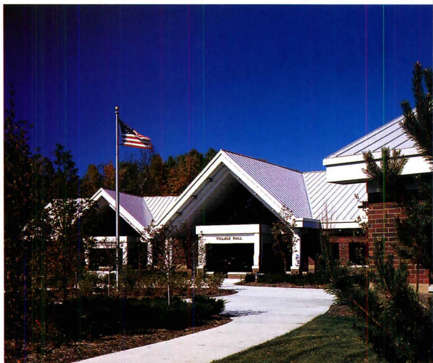
Orono City Hall Architect: Boarman Kroos Phister Rudin & Assoc. Roofing Contractor: Vohnoutka Roofing & Sheet Metal Co., Inc. Color: Sandstone
