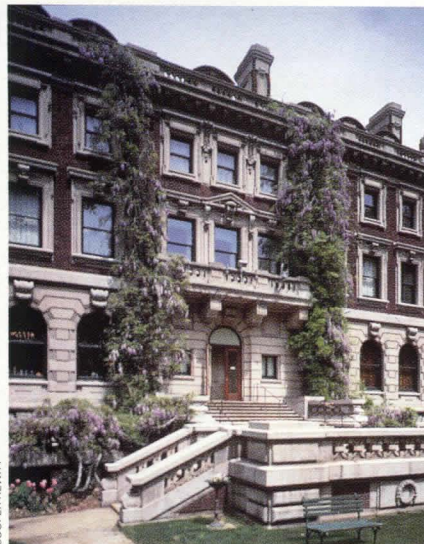
TERRACE: Existing layout bars disabled.
