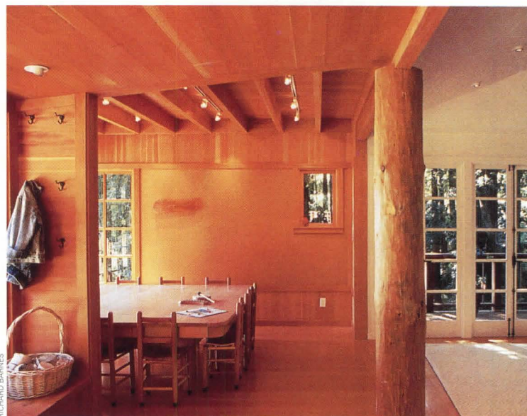
BUCKLEY SCHOOLHOUSE: Peeled log column was incorporated by Fernau and Hartman.
