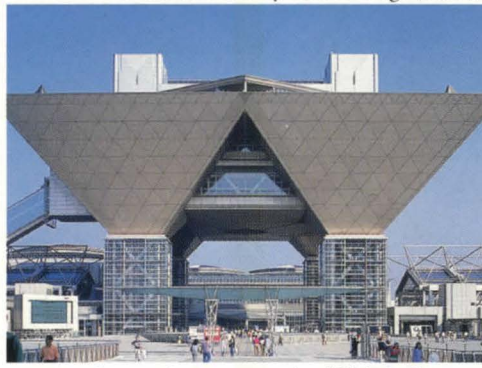
BIG SIGHT: Convention center on landfill (1996).
