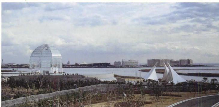
ABOVE: Taniguchi's octagonal entry pavilion at Sea Life Park Aquarium (left) contrasts with his sail-like structures marking shoreline of Tokyo Bay. FACING PAGE: Aluminum panels and steel mullions of Kasai Rinkai Viewpoint Visitors Center's curtain wall demonstrate Taniguchi's nested proportional systems.
