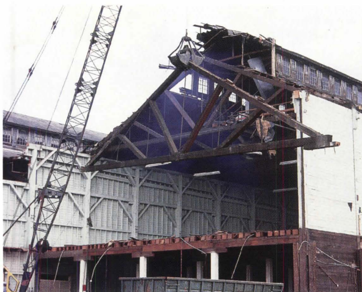
LONG-BELL LUMBER MILL: Millions of board feet were salvaged, including trusses.
