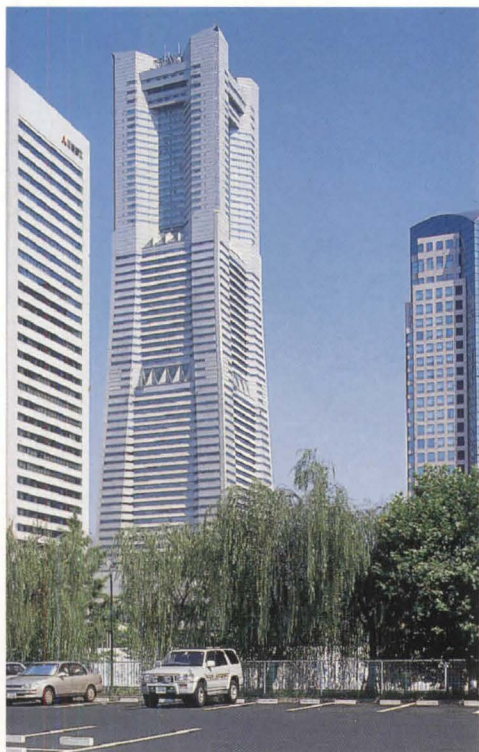
LANDMARK TOWER: Stubbins Associates’ Yokohama icon.
