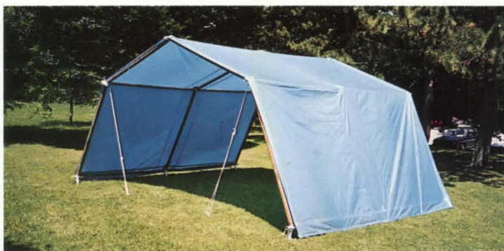
FACING PAGE: Shigeru Ban sits in his Paper Gallery (1994), built for fashion designer Issey Miyake. Chairs were also designed by Ban. ABOVE: Paper-tube-supported tents were designed for Rwandan refugees.
