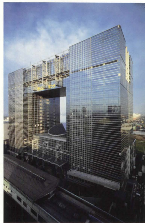
TOKYO TELECOM: HOK's Telecom Center (1996).
