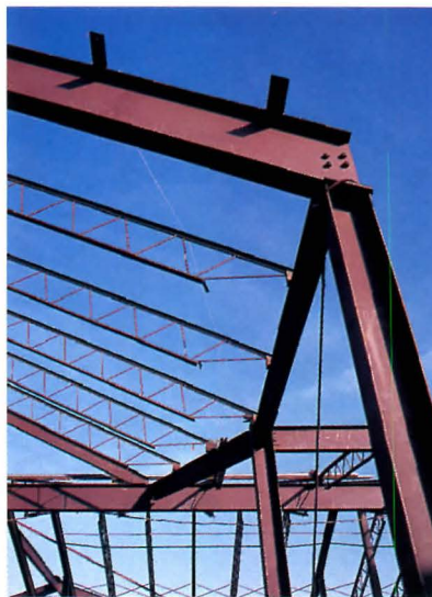
Sloped seat joists can be designed to fit almost any degree of pitch.
