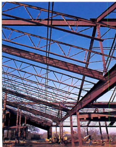
Sloped seat joists work in even the most complex customized framing jobs.
