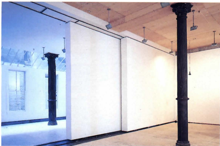
SLIDING WALLS: Subdivide interior for installations.
