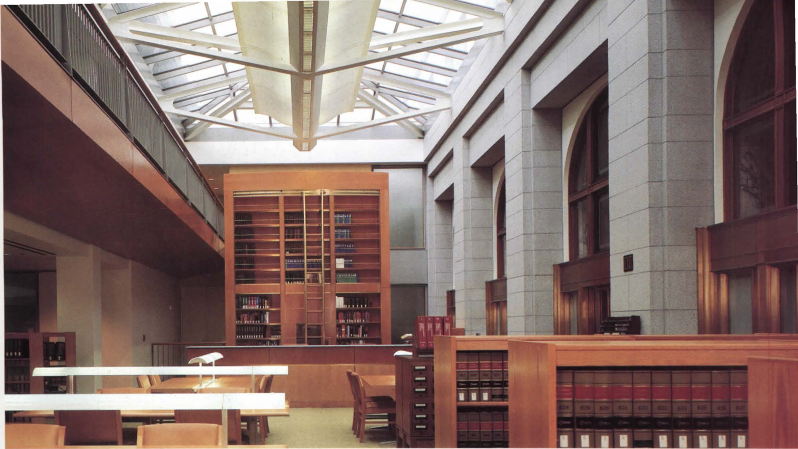
Law library's reading room stretches between monumental cherry bookcases containing seldom-used volumes. Steel web supporting skylight frames new walls and ties existing parts into single diaphragm. Extensive daylight-simulation testing determined frits of skylight glazing.
