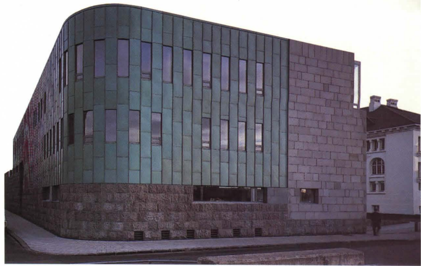
Cladding of copper, basalt, and gabbró wraps northwest corner of building (above). Solid basalt block anchors southwest corner, marking court's public entrance (below). Balcony above entrance is used for presidential inaugural addresses. Slotted windows illuminate offices of Supreme Court justices.
