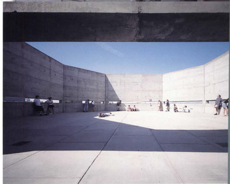
Concrete roof court (top), between octagonal planetarium and exhibition wing, will serve as a venue for future outdoor exhibits. Open to sky, star court on top of planetarium (above) offers panoramic view of Phoenix through continuous slots at children's height.
