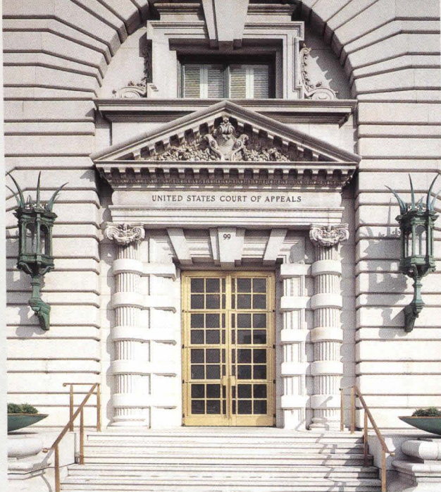
Granite was cleaned with mild soap-and-water solution. Bronze lanterns, replicas of designs for Palazzo Strozzi in Florence, were cleaned and outfitted with new electrical wiring.
