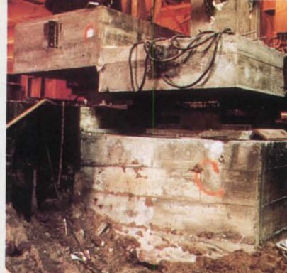
Court building floats on 256 friction pendulum bearings (above and below). Structural columns were cut at bases, lifted hydraulically, and fitted with concrete foundations. SOM studied three column-jacking options (bottom), but chose concrete for compatibility with old and new materials.
