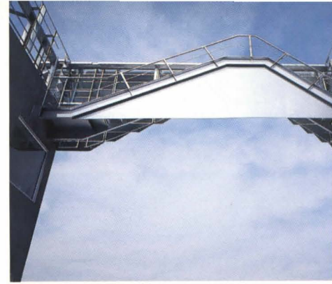
Steel bridges and stairs connect top level of north-facing wings, which house executive offices. Their intricacy displays skills of long-time Moss collaborator, steel fabricator Tom Farrage.
