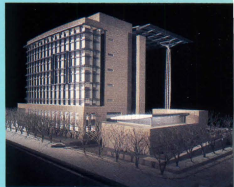
U.S. Courthouse in Las Vegas (left and above) embraces monumental plaza. Freestanding, 160-foot-tall column supports steel canopy.
