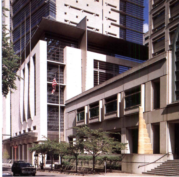
Steel canopy tops ground level of west facade to echo scale of adjacent Justice Center by ZGF. Two-story loggia and trio of ceremonial flagpoles demarcate court's main entrance.
