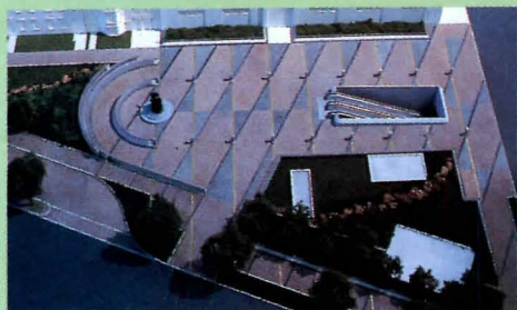
Devroux & Purnell's African-American Civil War Memorial sits atop Shaw Metro station.
