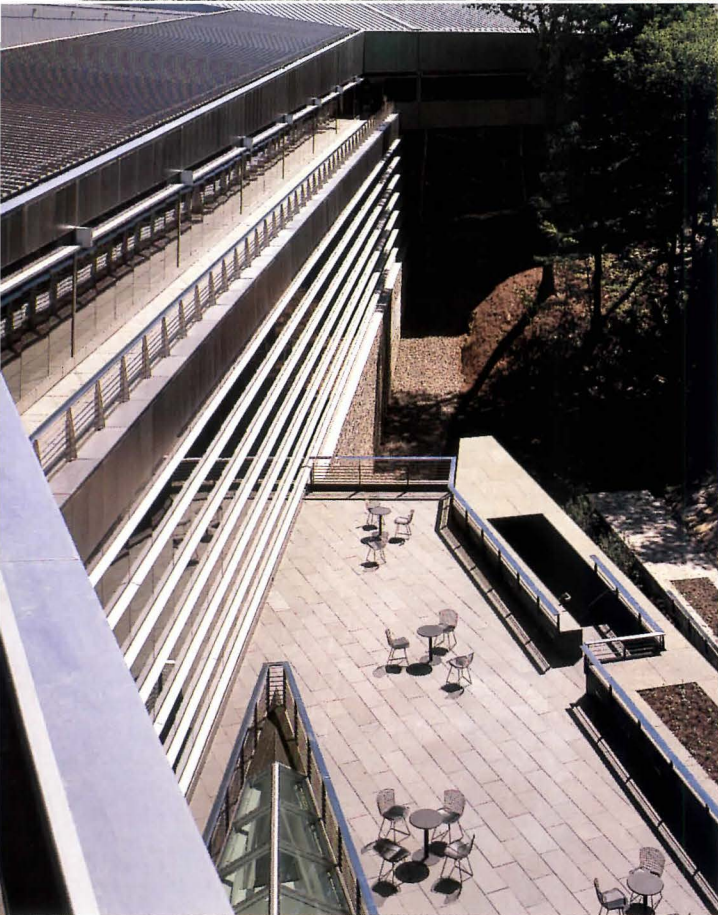
Like a Swiss Army knife, blades of IBM headquarters (top) unfold from building into surrounding woods, where landscaped parking lots follow contours of hillsides. Third-floor executive terrace on south facade (above) overlooks ground-floor terrace and ravine. Rear terrace (facing page), located off lobby leading to cafeteria, serves as company piazza.
