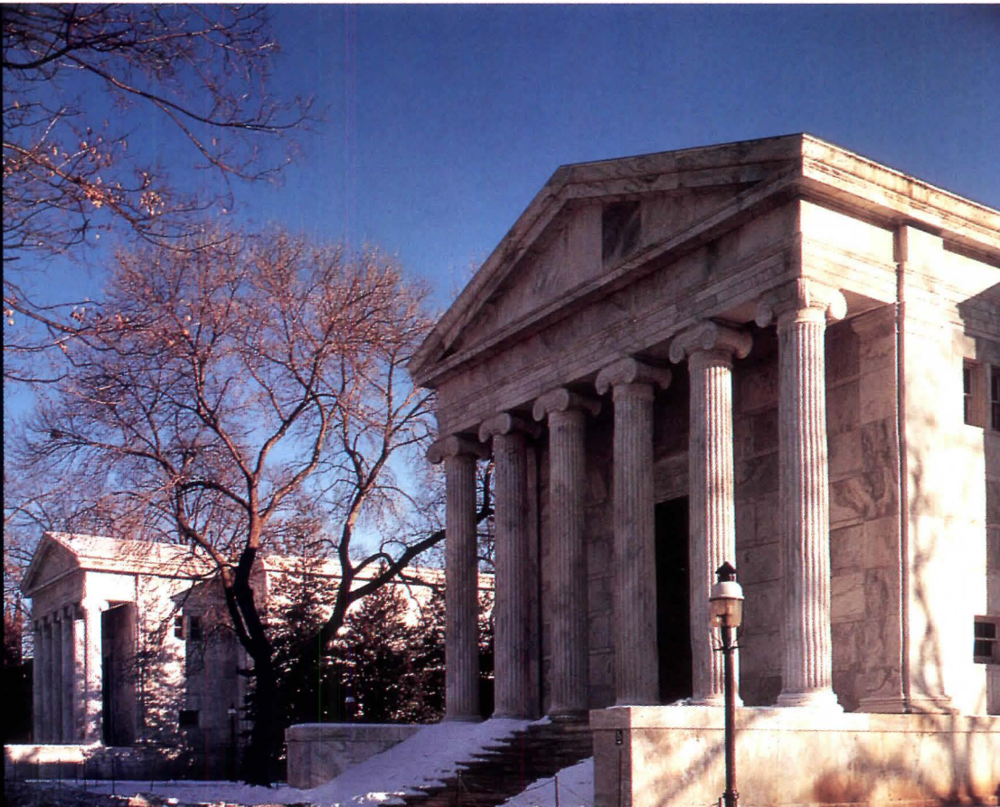
Cracks in 22-foot-long column shafts of Whig and Clio halls (right) were repaired with pinning process. Bases had to be replaced.
