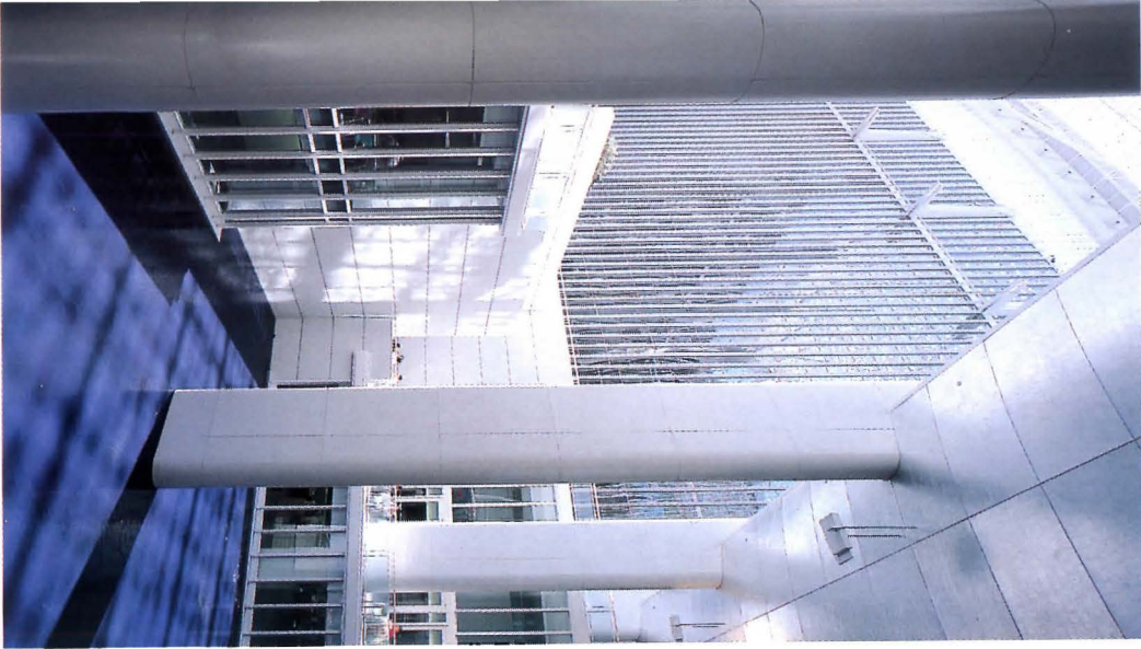
Concrete pilotis supporting north flank of offices extend into basement-level reflecting pool (left). Subterranean cafeteria and travel office flank light well and pool below atrium (right). Plans reveal pinwheel arrangement of offices around central atrium.
