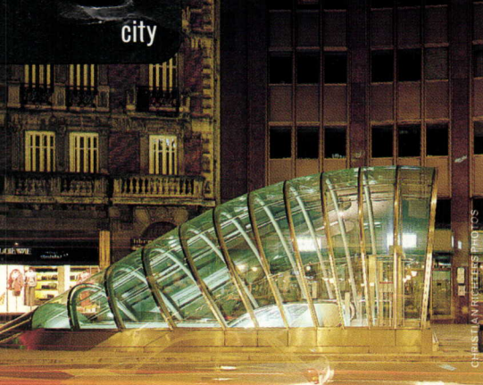
Norman Foster's new citywide subway system features glazed entrance canopies (above) and vaulted concrete platforms (right).
