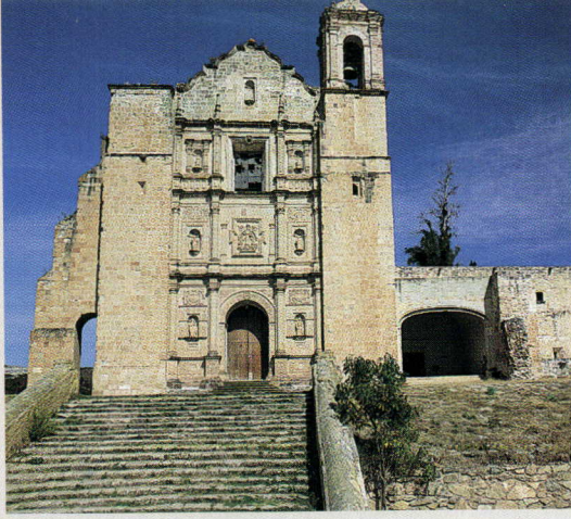
In Oaxaca, Mexico, a 22-meter-high retablo is being restored and stabilized by the Getty within the Church of Santo Domingo.
