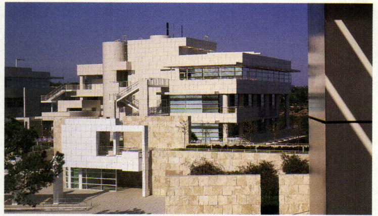
9 Cylindrical stair towers mark conservation building, seen from central courtyard.
