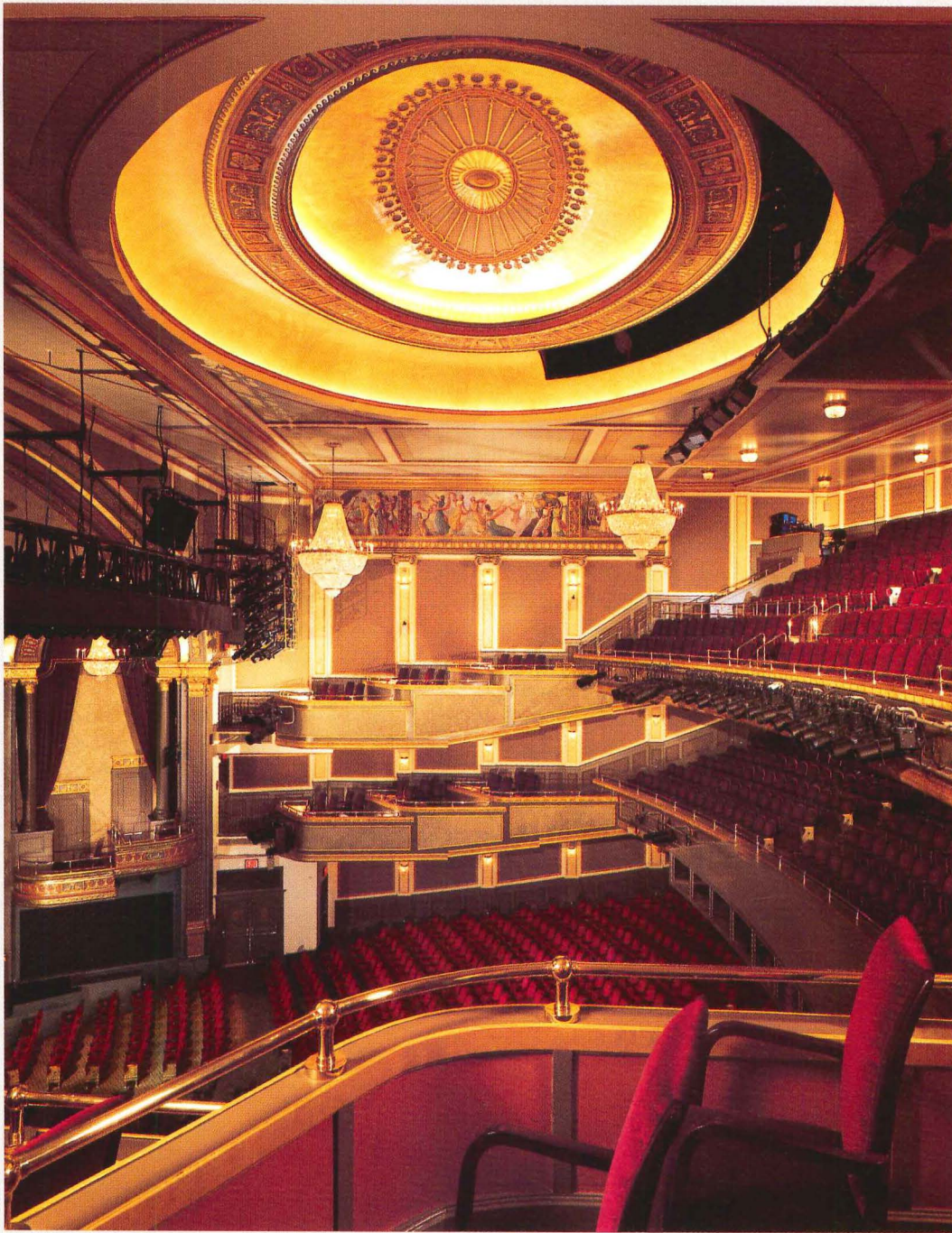
Conservators disassembled Apollo's proscenium arch (facing page, left) and elliptical dome and transferred them to New Jersey warehouse. New steel armature (facing page, center) was installed to rejoin dome. Lyric's dome (facing page, right) is a replica of damaged original. Reassembled and regilded Apollo dome (left) hovers over new 1,821-seat auditorium.
