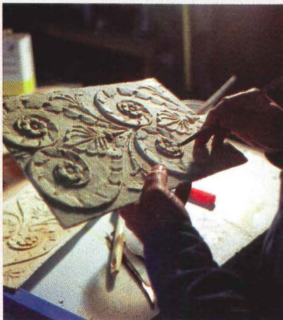
Plaster ornament from original box seating, proscenium arch, and sail vault (right) were refinished and replaced by hand.
