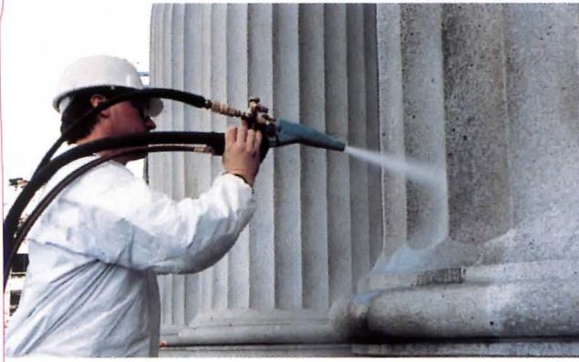
Low-pressure, rotating water spray mixed with fine, inert mineral powder cleans masonry. Brick and stone surface (above right) before and after treatment with JOS system.
