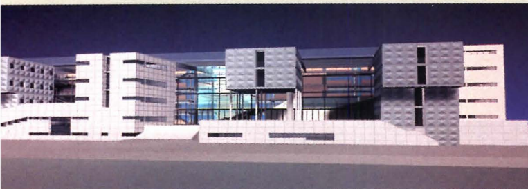
Marne La Vallée School of Architecture Champs-sur-Marne, France
