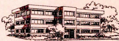
OFFICE BUILDING, 2-4 STORY Face brick with concrete block back-up and steel joists
