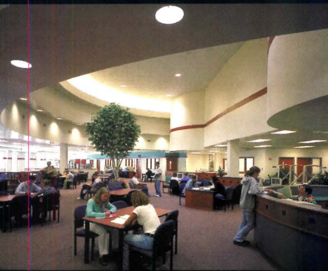
In media center of 400,000-square-foot Wayzata High School, architect Armstrong, Torseth, Skold & Rydeen specified costlier but more durable impact-resistant gypsum for perimeter wall and other areas affected by student traffic, but standard gypsum board for out-of-reach areas like curved ceiling elements.
