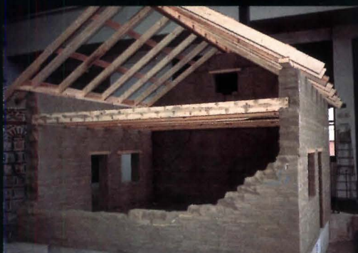
Adobe models built by Getty Conservation Institute allowed scientists to improve adobe's seismic stability. Model braced with steel (top) survived shaking table tests while reinforced model (above) collapsed.
