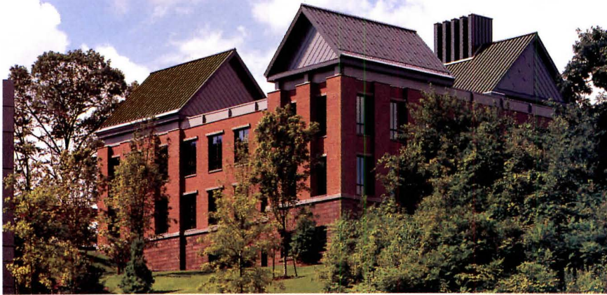
Light floods Duracell headquarters' main circulation spine (top left) through skylights. Lobby (top right) features veneers of renewable wood. Brick manufacturers used more than 5,400 pounds of scrap manganese powder from battery manufacturing process (which lends a dark hue) to create 400,000 bricks (above).
