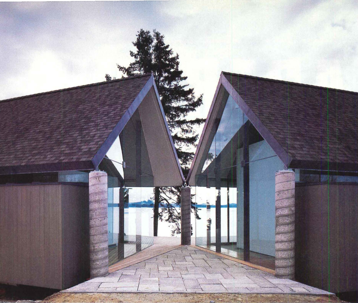
Peter Forbes-designed house (above) in Surry, Maine, completed in 1996, features fiberglass roof shingles, attic ventilation at roof peak, and cedar siding. Clerestory windows are protected by concrete pillar-supported overhanging eaves (matching detail, facing page, left). Forbes house under construction in Cape Cod, Massachusetts, includes tilt-up decks to protect windows (facing page, center) and (facing page, far left) and eave-ventilated attic.
