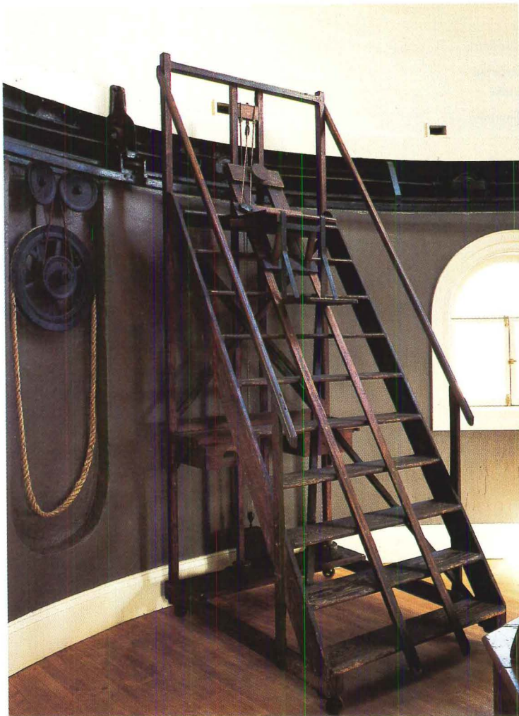
To left of newly refinished observer's chair (above left), hand-operated rope and pulley mechanism rotates dome. Room that contains meridian telescope (top right) includes new limestone clock pier (at right) lowered into place through ceiling hatch. In basement (above right), workers repointed masonry walls and telescope pier base (at right). During construction, team discovered original wood form (background) used to create basement and first-floor arches.
