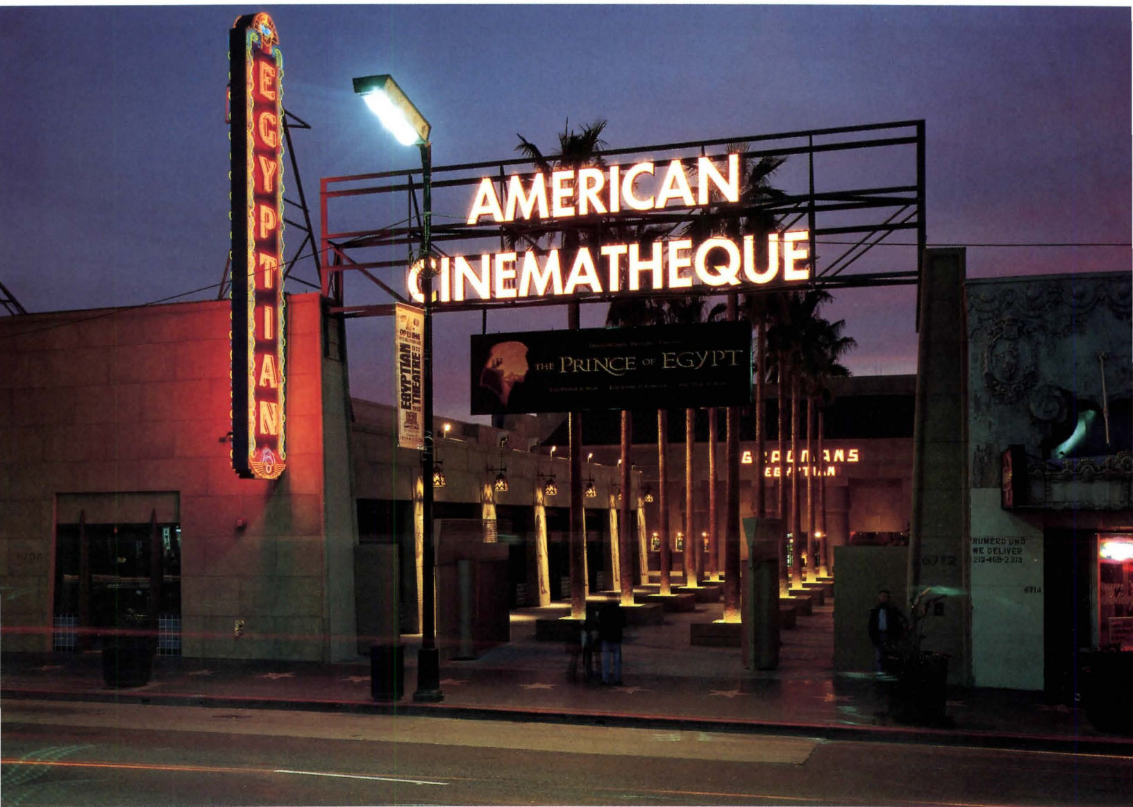
Egyptian motifs of restored plaster ceiling (facing page), including scarabs and pharoanic scepters, contrast with spare, technological esthetic of new auditorium enclosure. Ceiling ornament conceals historic pipe organ. Hodgetts + Fung planted palm allée in existing forecourt (above), creating open-air hypostyle that links Hollywood Boulevard with theater lobby. Flanking courtyard will be restaurant housed in renovated former shops.
