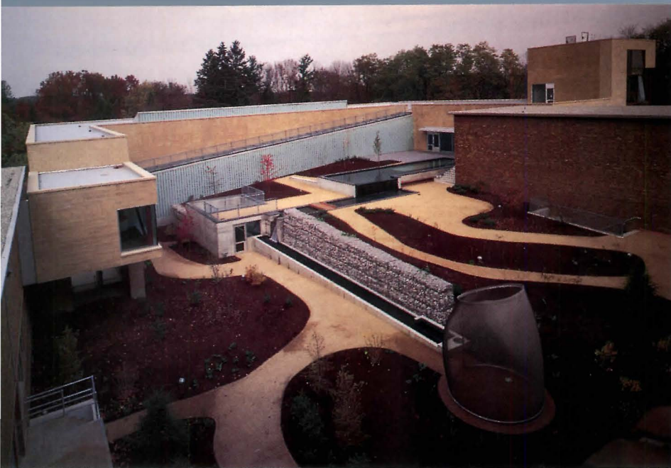
Science garden courtyard is located between Holl and Saarinen wings of science center (above); garden contains welded-steel House of Ice (at right) as well as concrete House of Vapor (at center) as part of demonstration of three physical states of water. Tiers of pools (below and facing page) demonstrate water in liquid state; glass block bottom of uppermost pool (facing page, at right) functions as skylight to gallery below.
