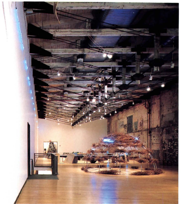
Light flows into gallery in Building 4 (left) through clerestory . To provide clear spans in galleries, architect cut existing wood columns (right), transforming them into king-post trusses by adding steel plates and lateral ties. Exterminators treated timbers with borate to prevent structural deterioration due to the presence of fungi—a common problem in mill conversions.
