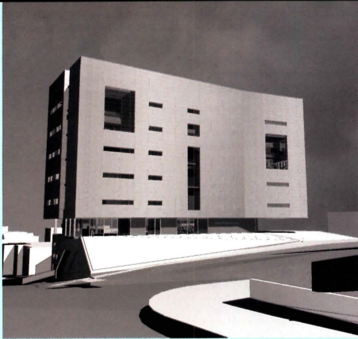
Large openings in limestone-clad south facade of Southern Poverty Law Center (above left) demarcate libraries and team meeting areas. In contrast, glazed north facade (above right) allows daylight open-office area. Concrete plinth mediates sloping site and creates public plaza. Bipartite composition (plan) segregates office and support functions. Eastern end of building splays to preserve views between memorial (axonometric, at left) and Dr. King Memorial Baptist Church (axonometric, at right).
