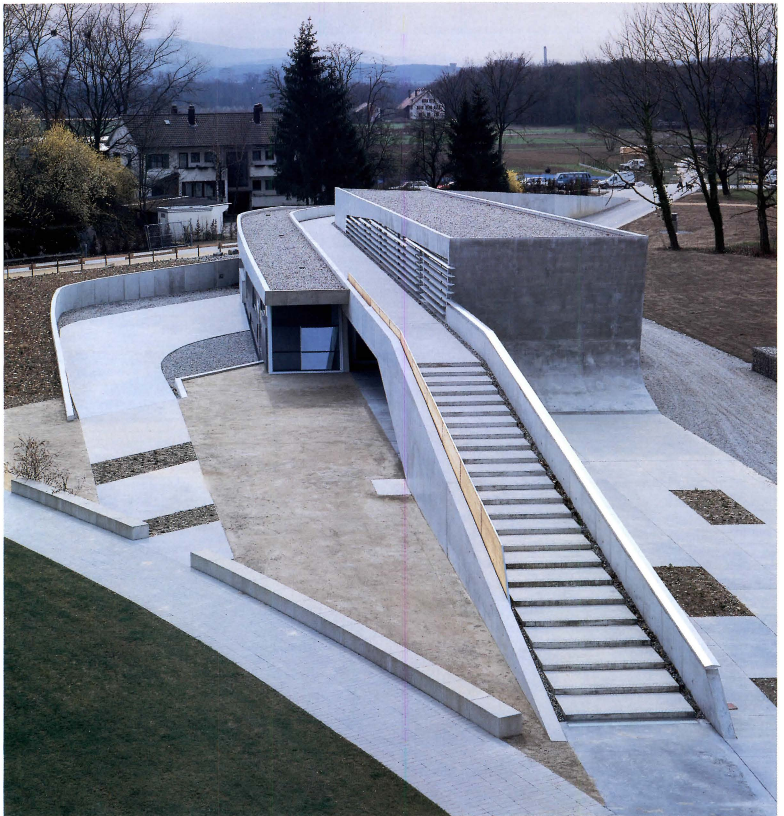
Shallow steps ramp up from north side of garden to rooftop terrace (above), which forms pedestrian circuit to second-floor gallery. To right of stairs is double-height volume of exhibition space; to left is smaller café flanked by outdoor dining terrace.
