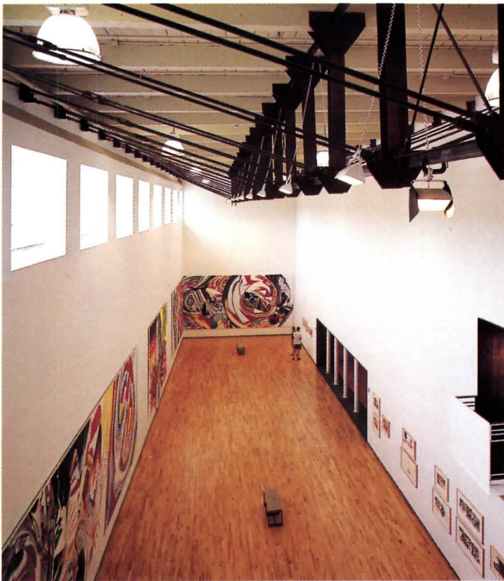
Light flows into gallery in Building 4 (left) through clerestory . To provide clear spans in galleries, architect cut existing wood columns (right), transforming them into king-post trusses by adding steel plates and lateral ties. Exterminators treated timbers with borate to prevent structural deterioration due to the presence of fungi—a common problem in mill conversions.
