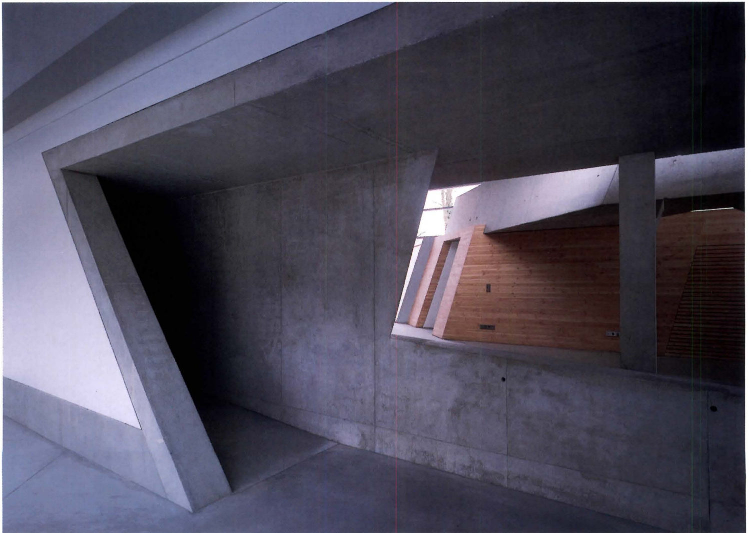
LANDSCAPE FORMATION ONE, WEIL AM RHEIN, GERMANY CLIENT: Weil am Rhein State Flower Exhibition ARCHITECT: Zaha M. Hadid with Patrik Schumacher, London and Mayer Bährle, Lörrach, Germany—Markus Dochantschi (project architect), Oliver Domeisen, Wassim Halabi, James Lim, Garin O'Avazian, Barbara Pfenningsdorf (project team) ENGINEER: Dr. Ing. L. Martino (structural) COST: $2.1 million PHOTOGRAPHER: Christian Richters, except as noted
