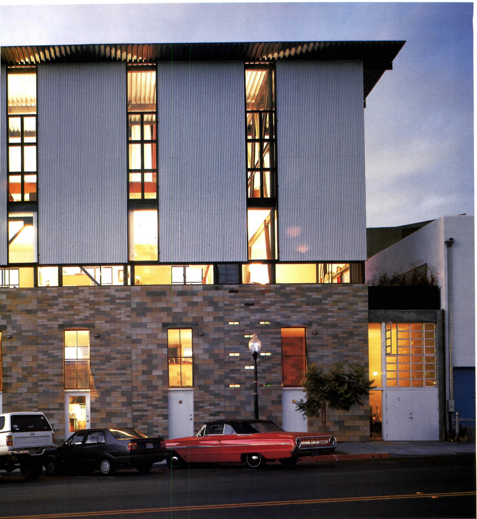
On northern street front, Merrimac (above) rises from base of multicolored brick, perforated by glass block. Doors lead directly to individual double-height studios; windows above doors look through to mezzanine level. Corrugated metal siding wraps upper floors.
