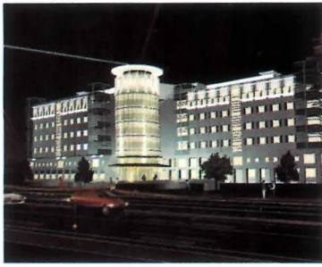
Ellerbe Becket's Center for Rehabilitative Medicine in Moscow.
