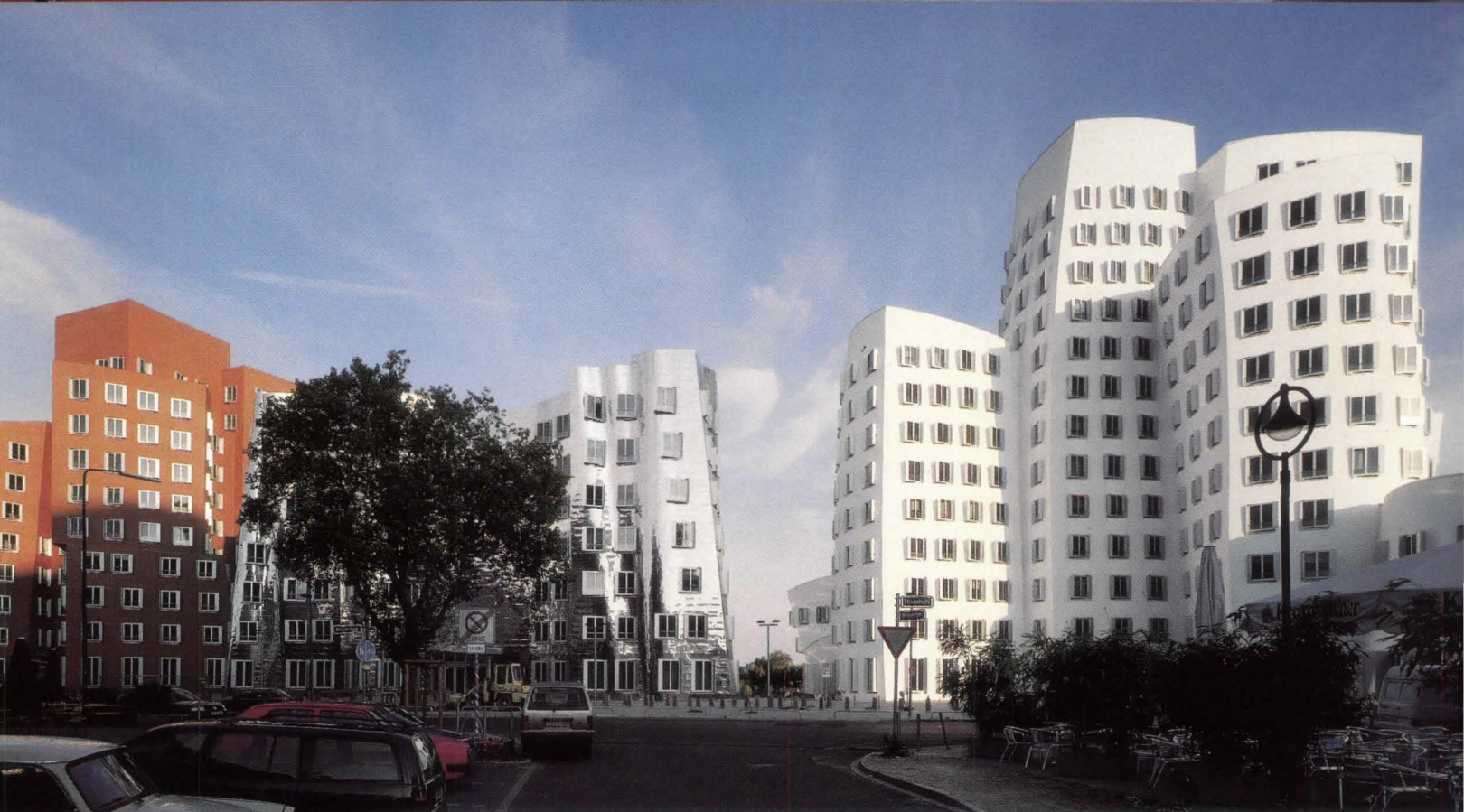
Gehry's arrangement of towers (above) frames views from the city across the Rhine River. His positioning also creates small-scale urban plazas (top right) between the towers. Rather than customizing each window to fit the buildings' irregular surfaces, Gehry inserted standard windows into deep frames that project out of the façades and into each office (top left).
