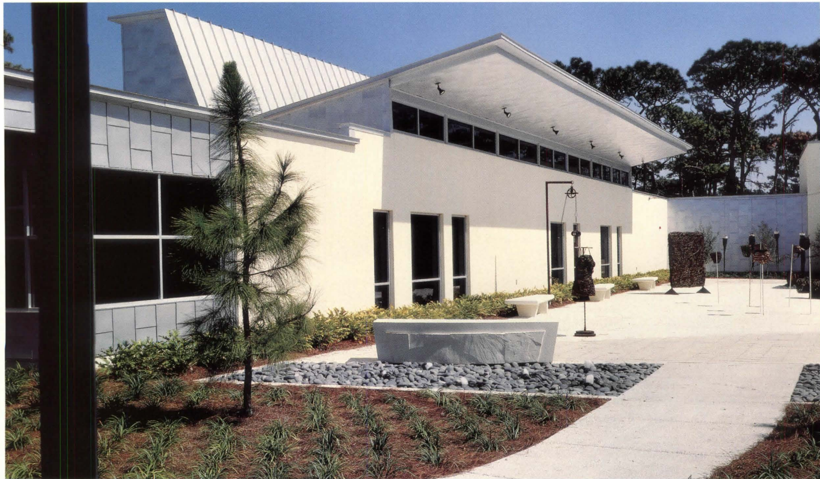
Tucked high up under a canopy on the south-facing side of the GCAC's administration wing, a bar of windows allows natural light into the office spaces without creating too much heat gain. A few larger openings at ground level look out onto the sculpture garden that sits between the wing and the galleries.
