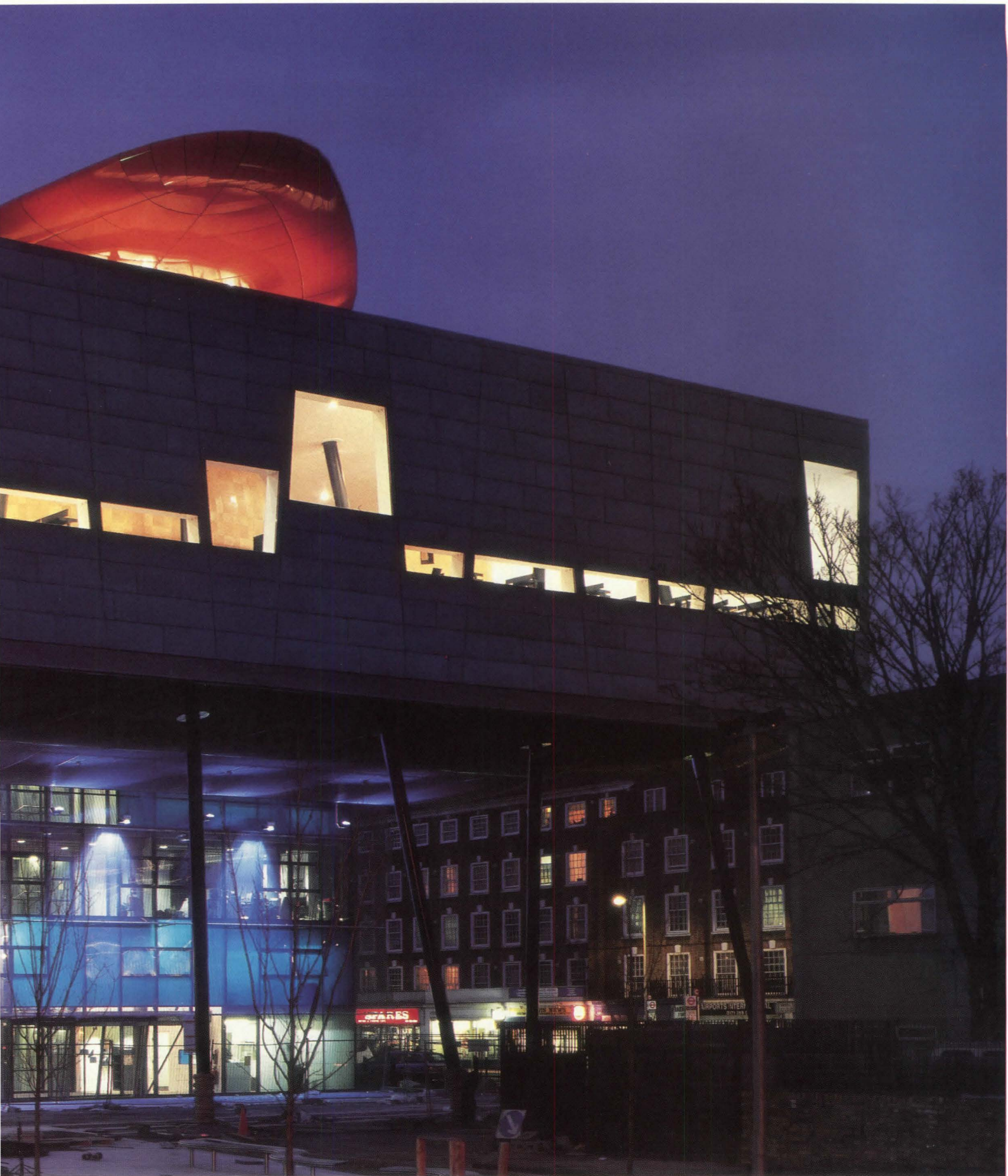
aluminum “canopy,” powder-coated in glossy orange, projects from the roof to provide additional shading and animate the roofline. Suspended floodlights cast a blue glow at night.
