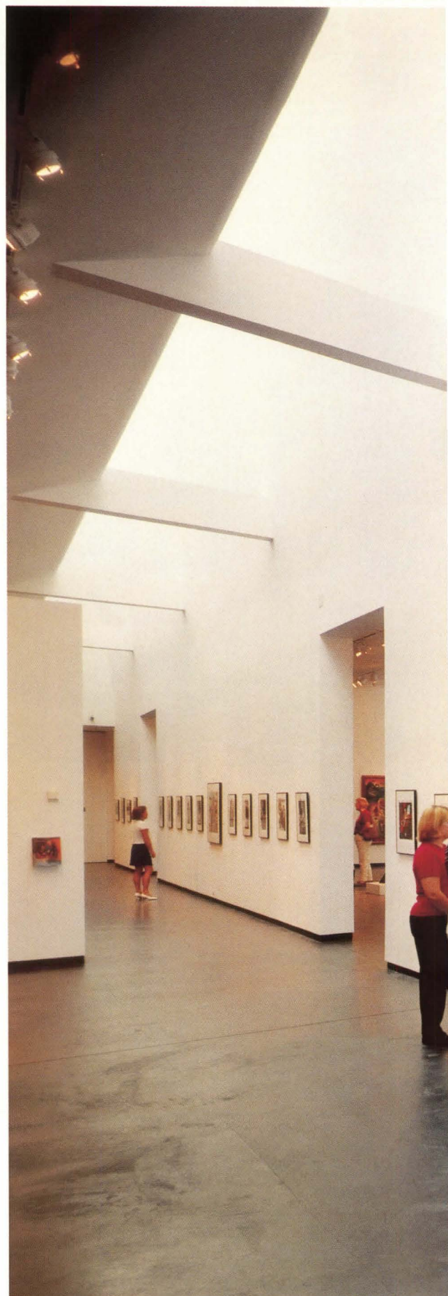
The galleries sit in three parallel bars (above and facing page), and are lit primarily with sunlight diffused by curved baffles set perpendicular to the walls. The aluminum cladding on the
