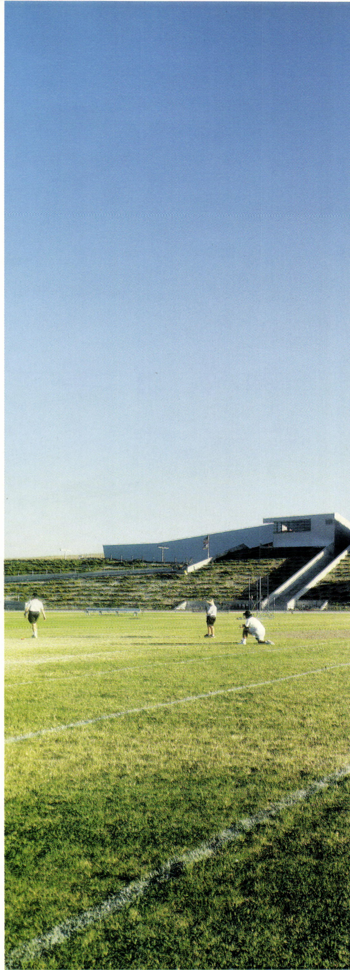
SITE WORK Three classroom wings cantilever over the lower playing fields (facing page, at right). Staircases (top) cut into the hillside and connect the school to the playing fields. A ramp (above) winds down from the library and administration block.
