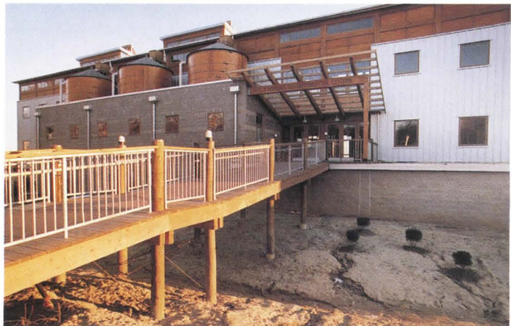
The building's parking area channels runoff away from the bay (top). Rainwater collects in cisterns and is used for sprinkler systems, sinks, and laundry (above).
