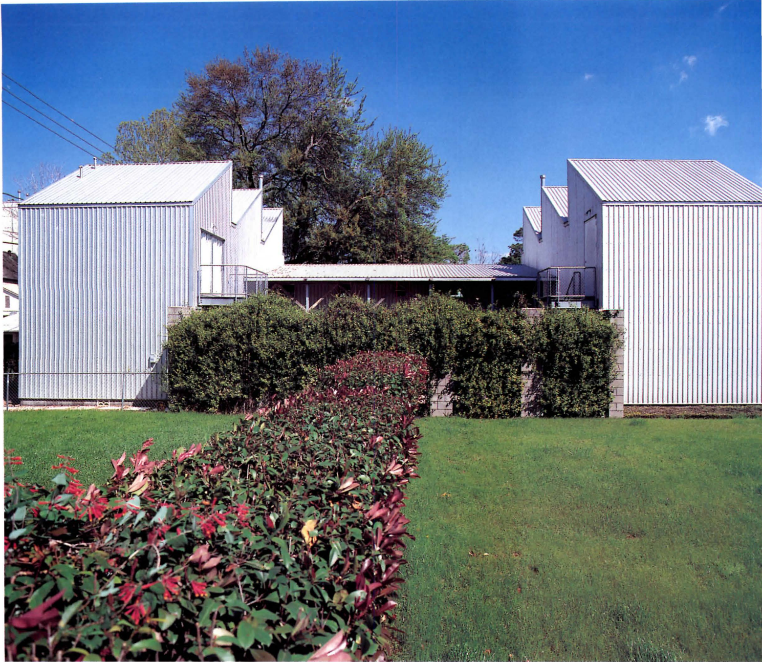
Taft built to the setback line, organizing the house internally around a central courtyard (above). The sawtooth roof of the two double-height wings incorporates light monitors that illuminate the studios within; an exterior metal stair (facing page, top) provides the only access to one of the studios.
