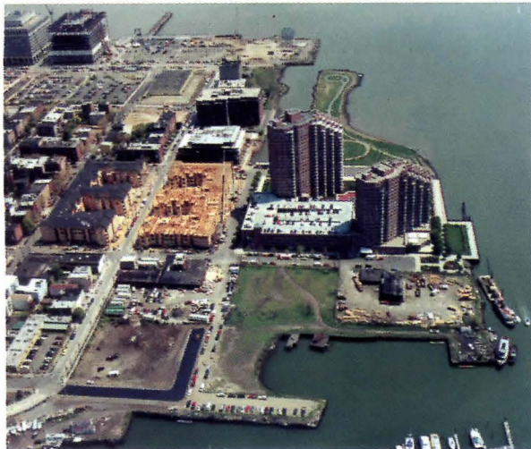
Brownfields, like this along the Jersey City, New Jersey, waterfront, can become prime real estate parcels.
