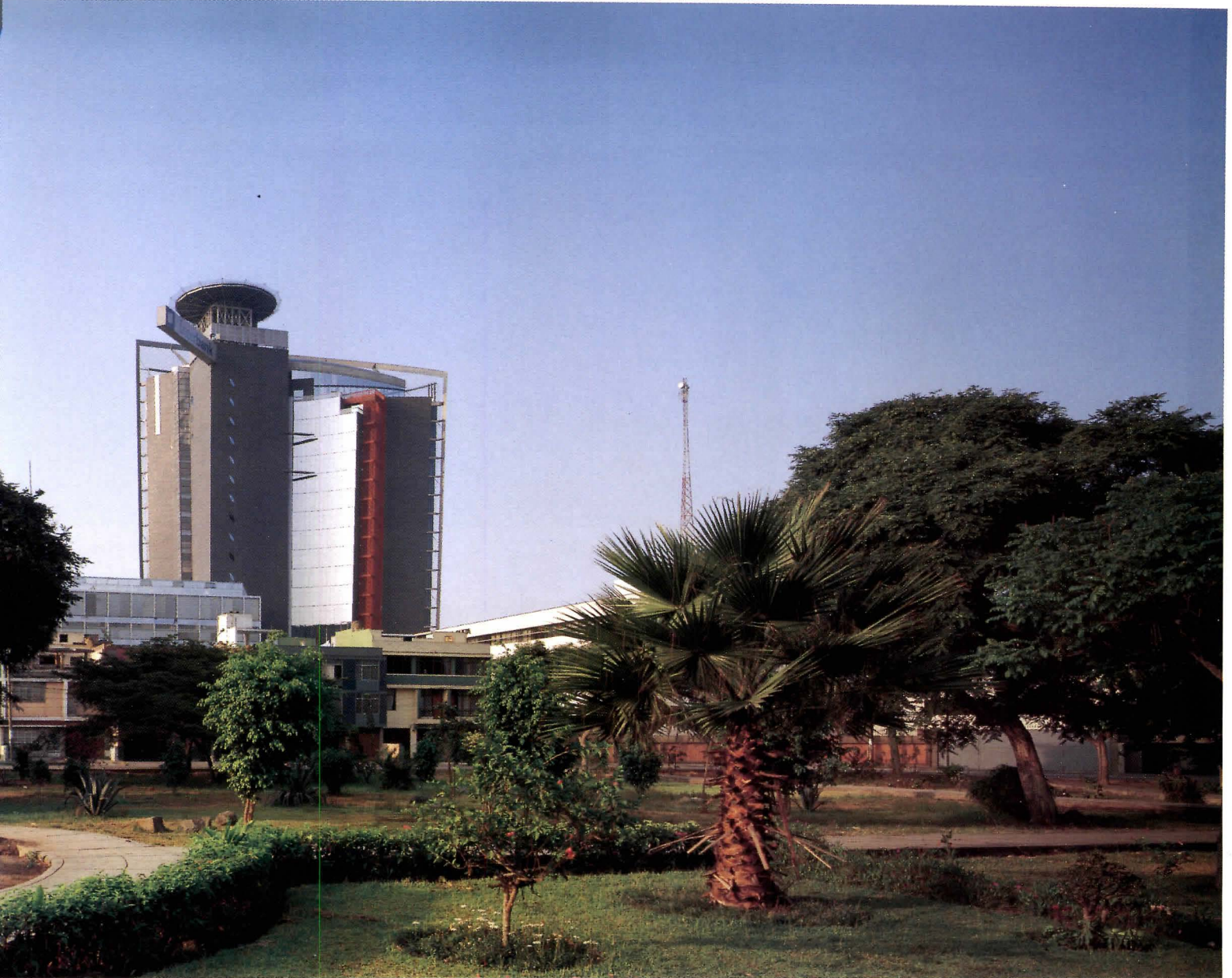
The tower's northern façade overlooks a much less hectic setting—a low-rise residential district and a park. The block-like service core with elliptical windows (above, at left) and a bright orange emergency-egress stair frame a strip of glass curtain wall.
