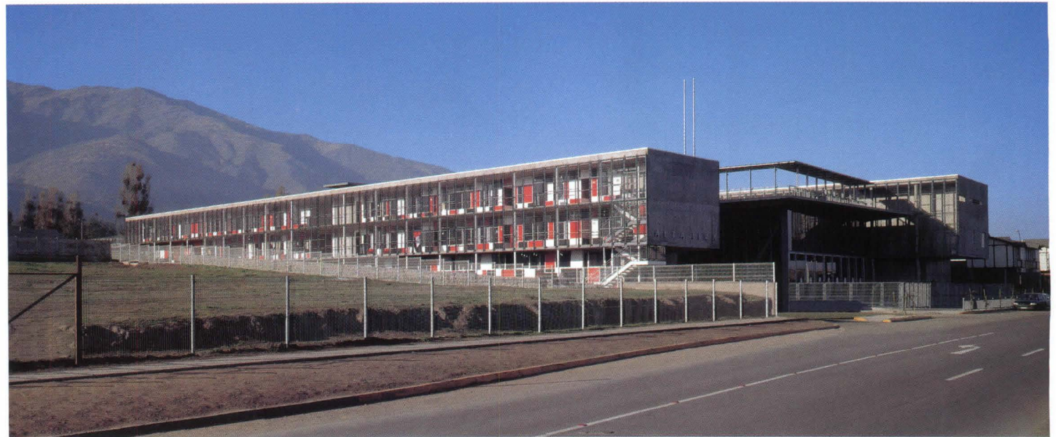
A student at Mathias Klotz's Colegio de Altamira (preceding spread) peers through a skylight in the surface of the playground to a gym below. The two long bars that hold classrooms flank a glazed gymnasium and are clad in vertical strips of pine on their respective southern sides (top). On the northern—and in the southern hemisphere, sunny—side of each of these bars, colorful corridors enclosed only by metal mesh (center) provide access to the classrooms. The gym's roof is also a sloping playground (bottom).
