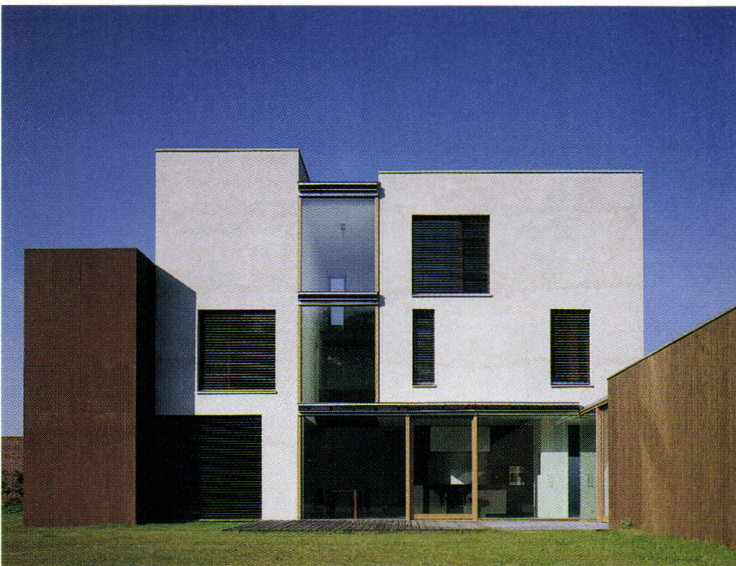
2B SOUTH FAÇADE
