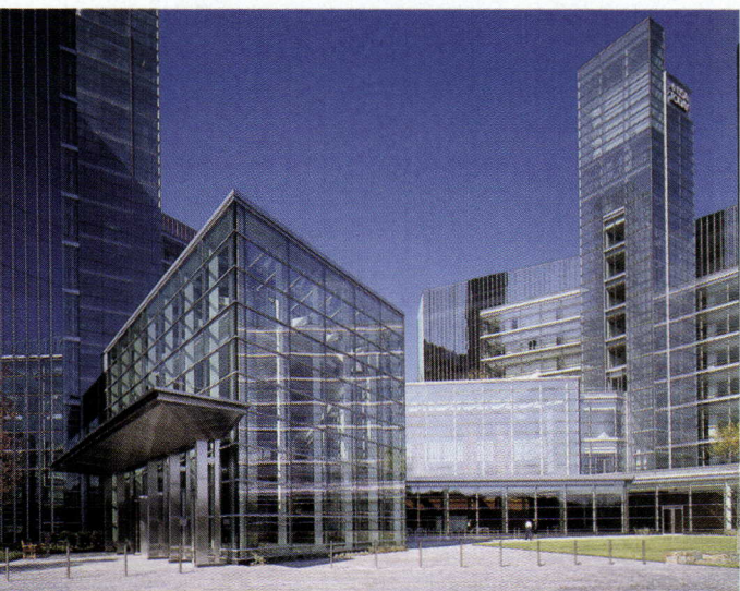
A spectacular mirage takes shape as glass-finned curtain walls blur the masses of KPF's Gannett/USA Today Headquarters (top). A parking garage (center) which will eventually be covered in ivy, keeps cars from dominating the building's parklike setting. The U-shaped building's inward-facing façades (bottom) open onto a reflecting pool, parkland, and jogging paths leading ultimately to a ball field at the far end of the site. Rooftop terraces and corridors (facing page) encourage social life in the building.
