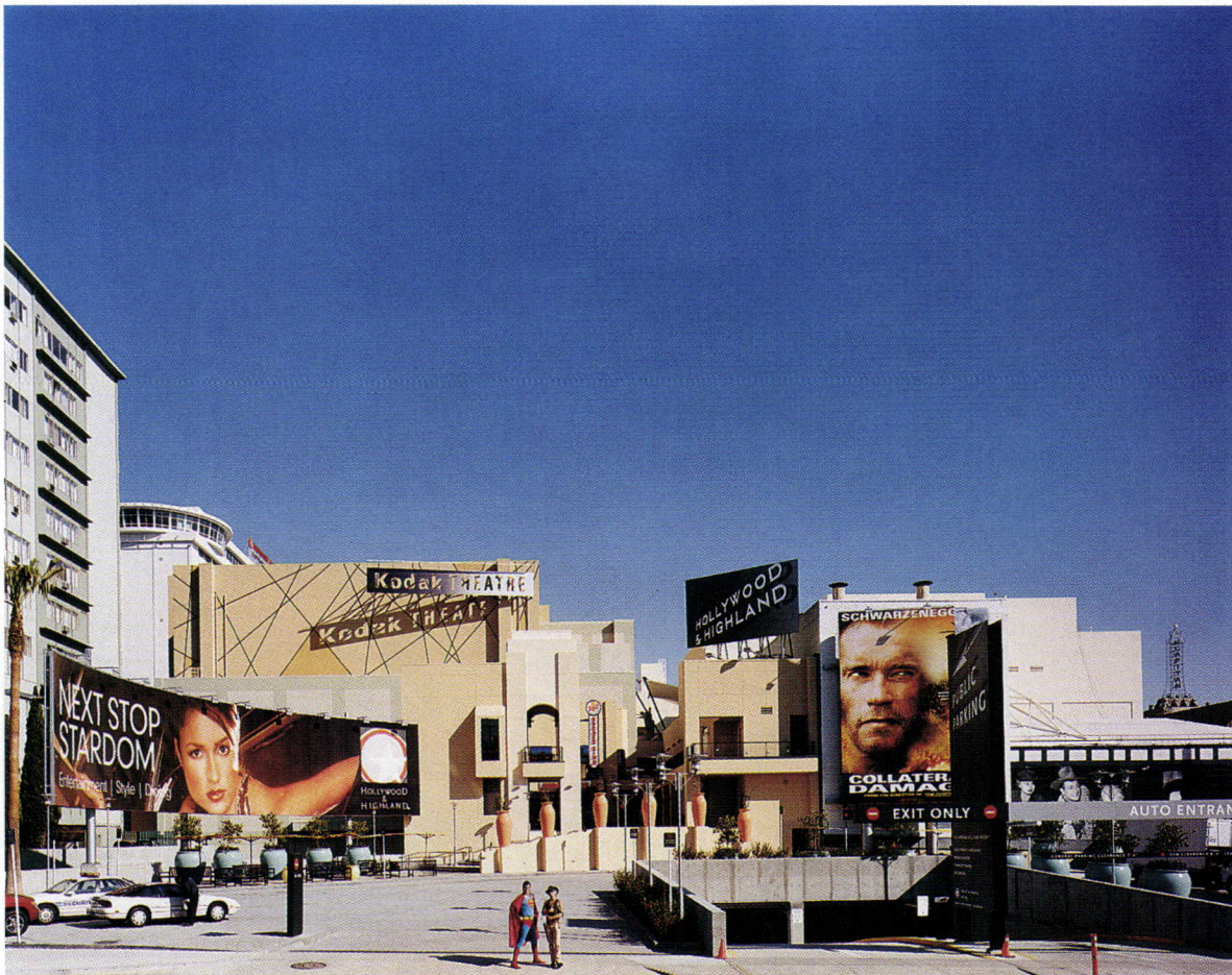
A side entrance to the complex, along Orange Street, incorporates two enormous billboards, “shadow” signage designed by Sussman/Prezja, and the entrance to a 3,000-car underground garage (above). The round form of a rooftop restaurant sits above a 640-room Renaissance Hotel that is part of the complex (at left).
