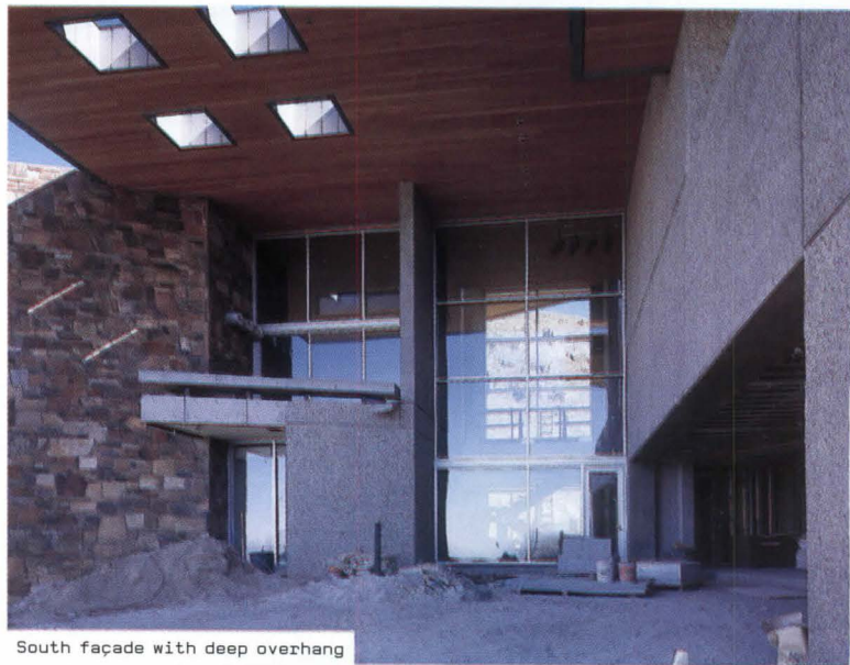
South façade with deep overhang
