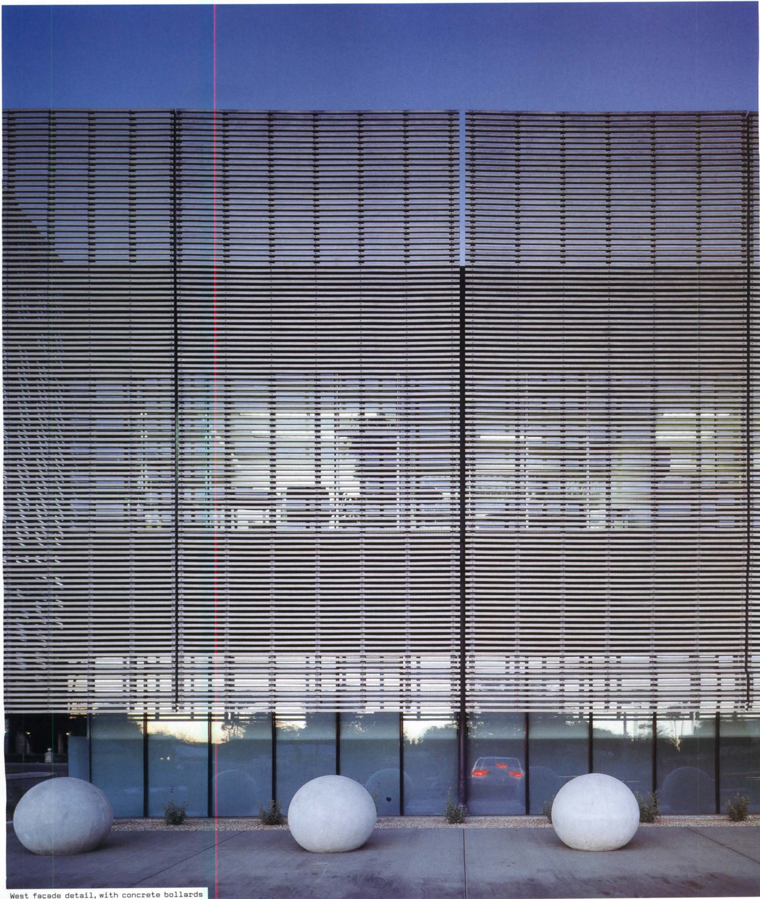
West façade detail, with concrete bollards
