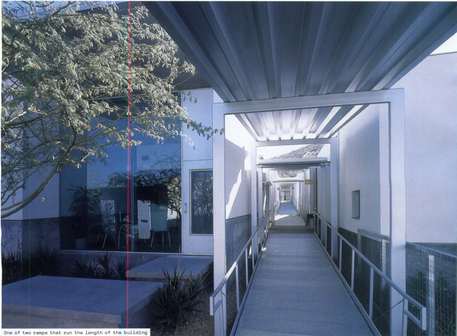
One of two ramps that run the length of the building
