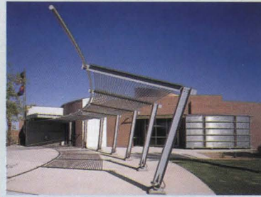
tempe police substation / 1995
