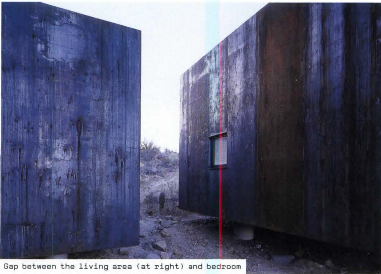
Gap between the living area (at right) and bedroom
