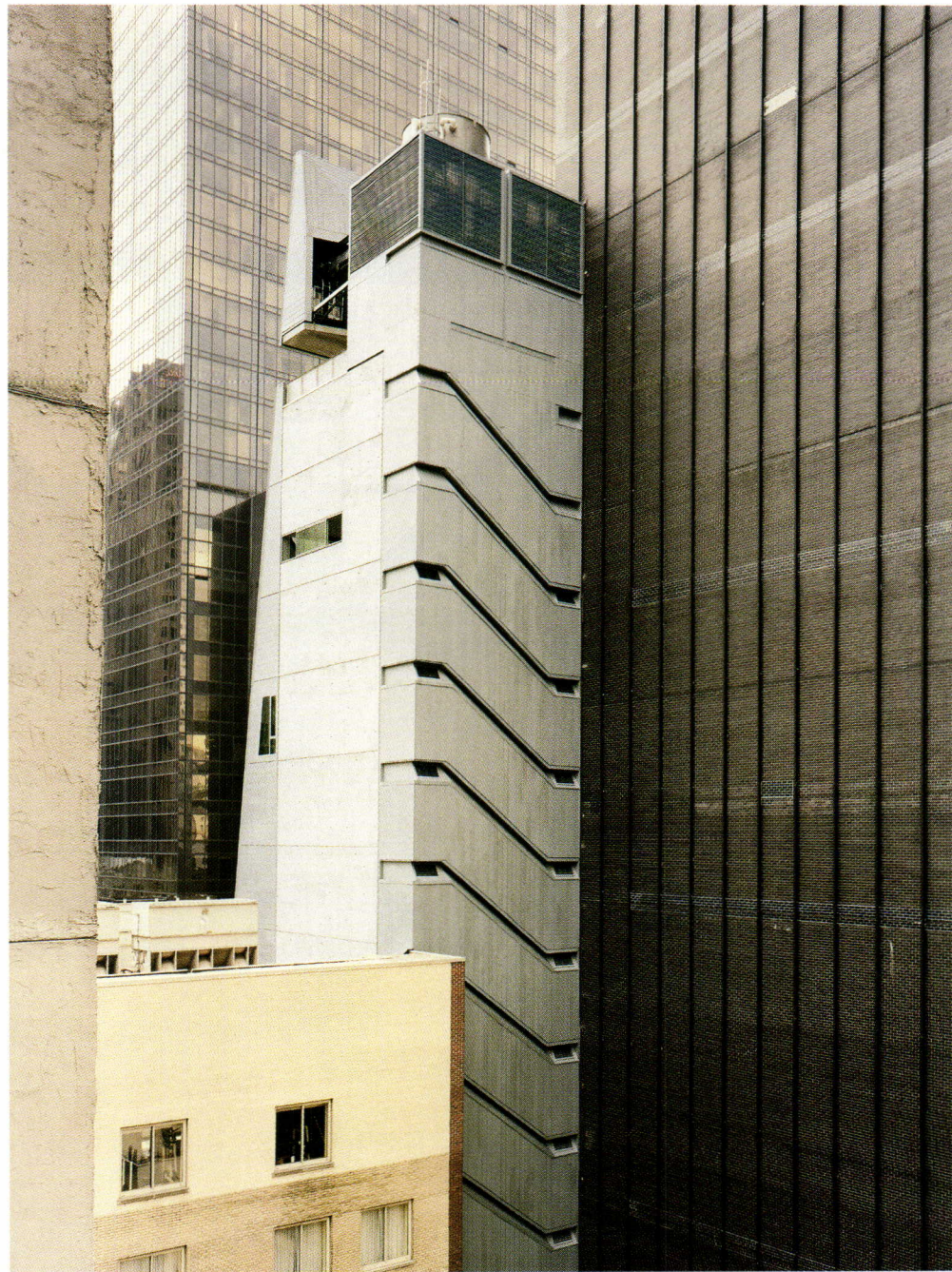
Slit staircase windows delineate the building's rear, north façade (above); while Abraham's vaguely anthropomorphic pattern of volumes and openings distinguish the north, entrance façade on East 52nd Street (facing page).
