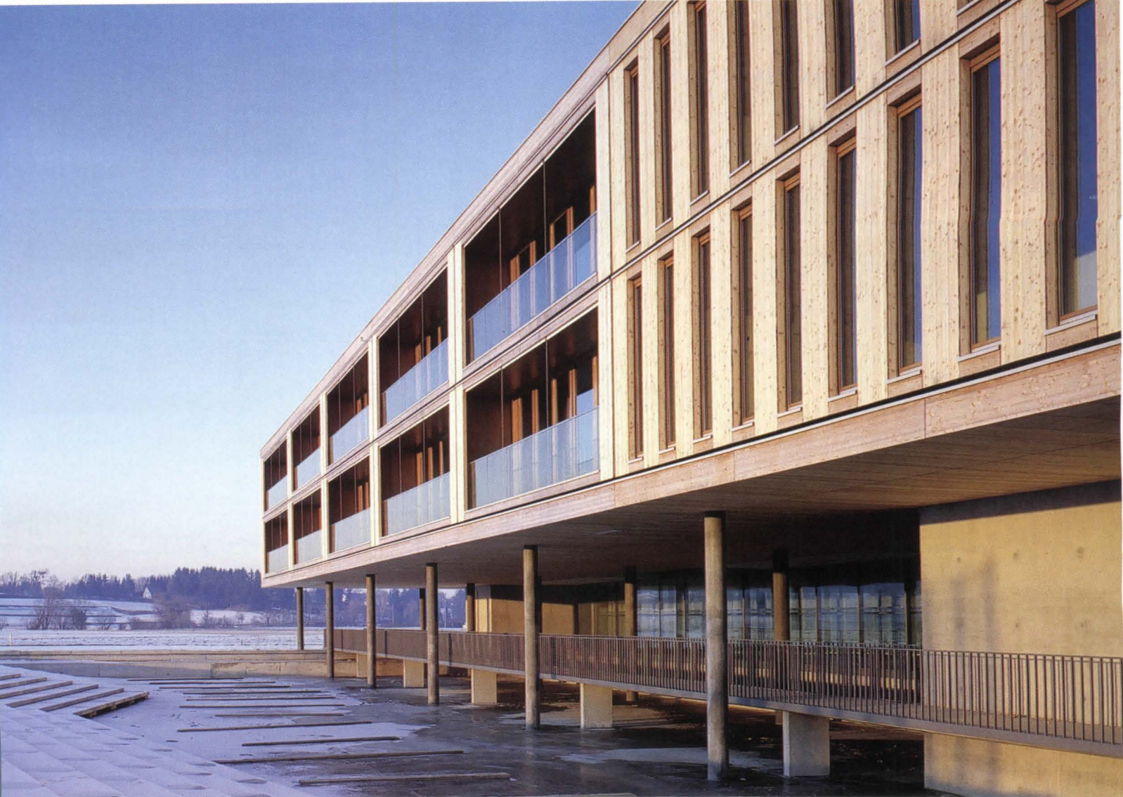
Located on the edge of the town of Markt Indersdorf, the grade school seems to float above its meadow site (facing page), freeing the ground level for play, sports, and socializing. The school's proximity to the flood-prone River Glonn drove the decision to elevate the structure on columns and to use concrete for the ground level, which contains the gymnasium and recreation hall. The architects chose wood cladding for the upper volume (above), in response to the rural surroundings.
