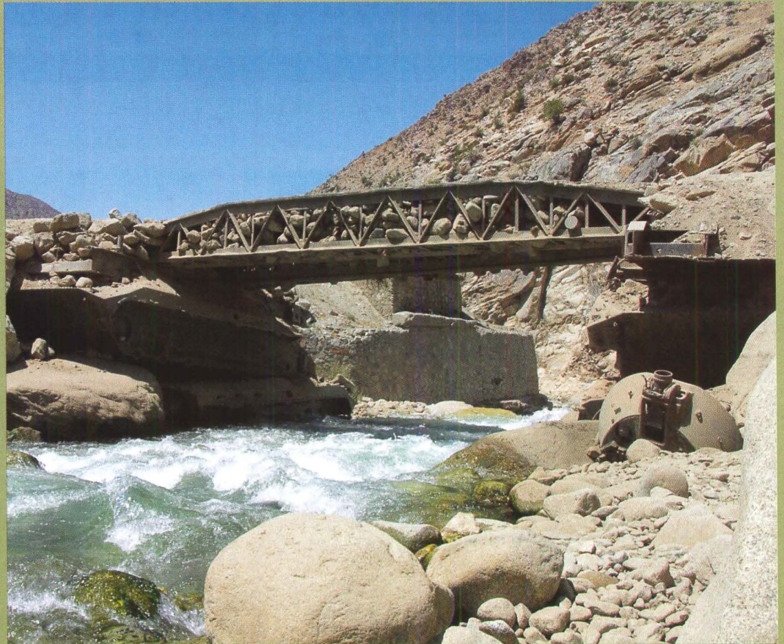
After years of war, Afghans have learned to use the materials available to them: Old tanks support a bridge (right), while stacked, spent shells form the wall of a shelter (lower left).
