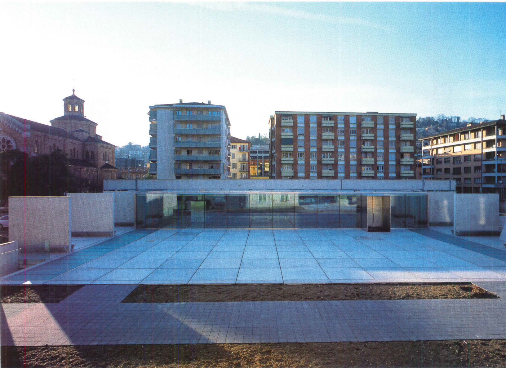
Glass-covered strips on either edge of the auditorium's plaza (above) provide natural light to the below-ground hall by day and are illuminated from below by night. The building's above-ground pavilion shelters a double-height lobby area (facing page).
