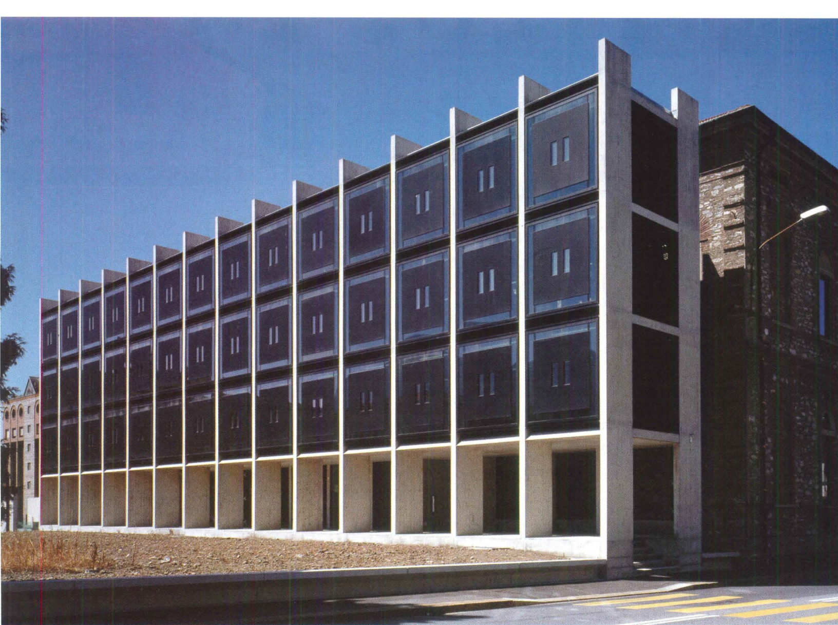
For the university's new library, architects Michele and Giorgio Tognola added a thin, façadelike structure, covering the open end of an existing U-shaped building (above). Inside, a row of study carrels is pushed against the building's outer wall, making use of natural light for reading (facing page).
