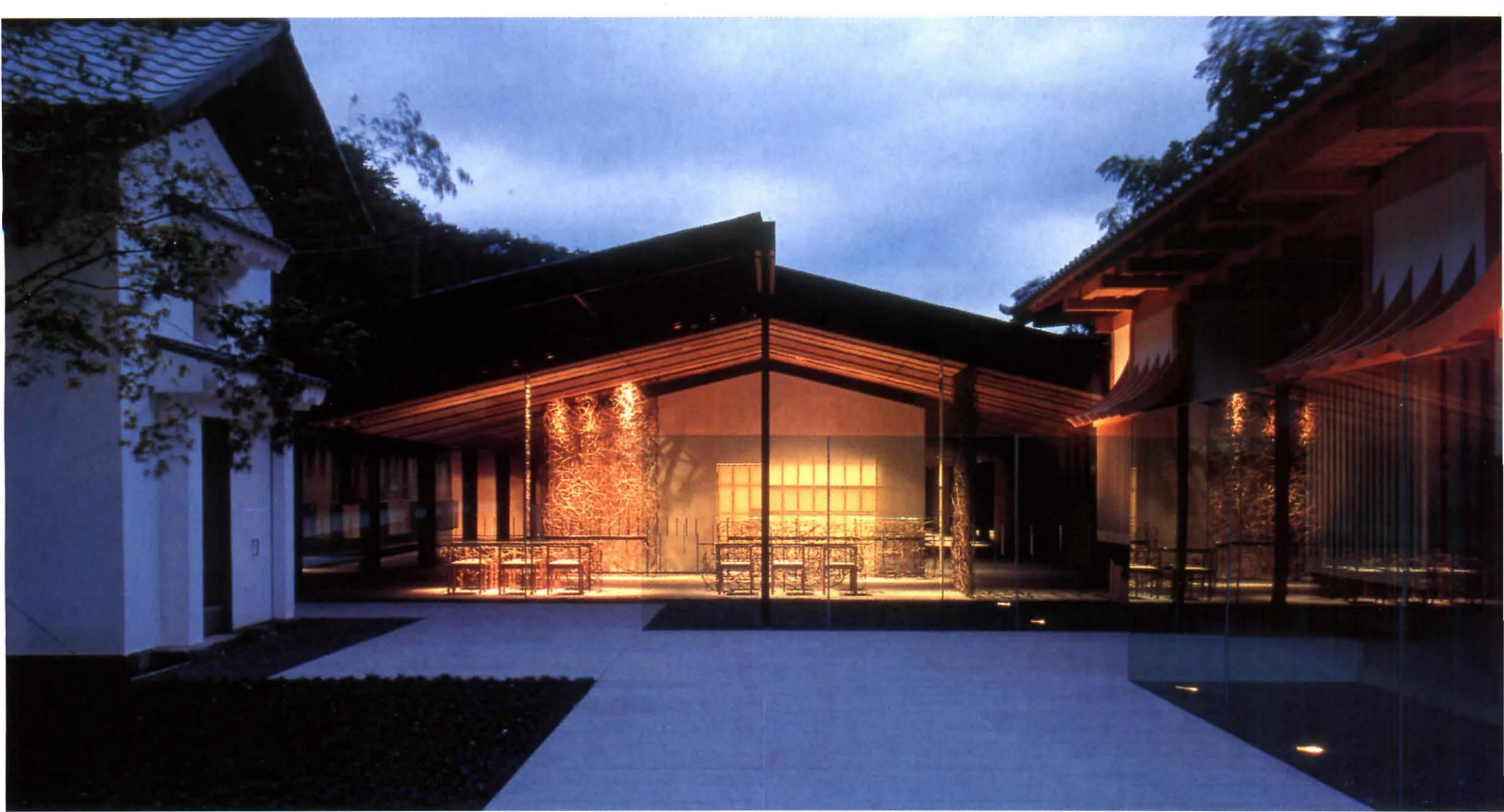
Down the road from the Stone Museum, the Nasu History Museum again demonstrates Kuma's adeptness in applying natural materials. Semitransparent panels made of rice straw adhered to aluminum mesh provide shade from direct sunlight (below). Vines collected from the local countryside provide a backdrop for the entry hall (above); ornamental logs attached to the roof also reference the local vernacular (facing page).
