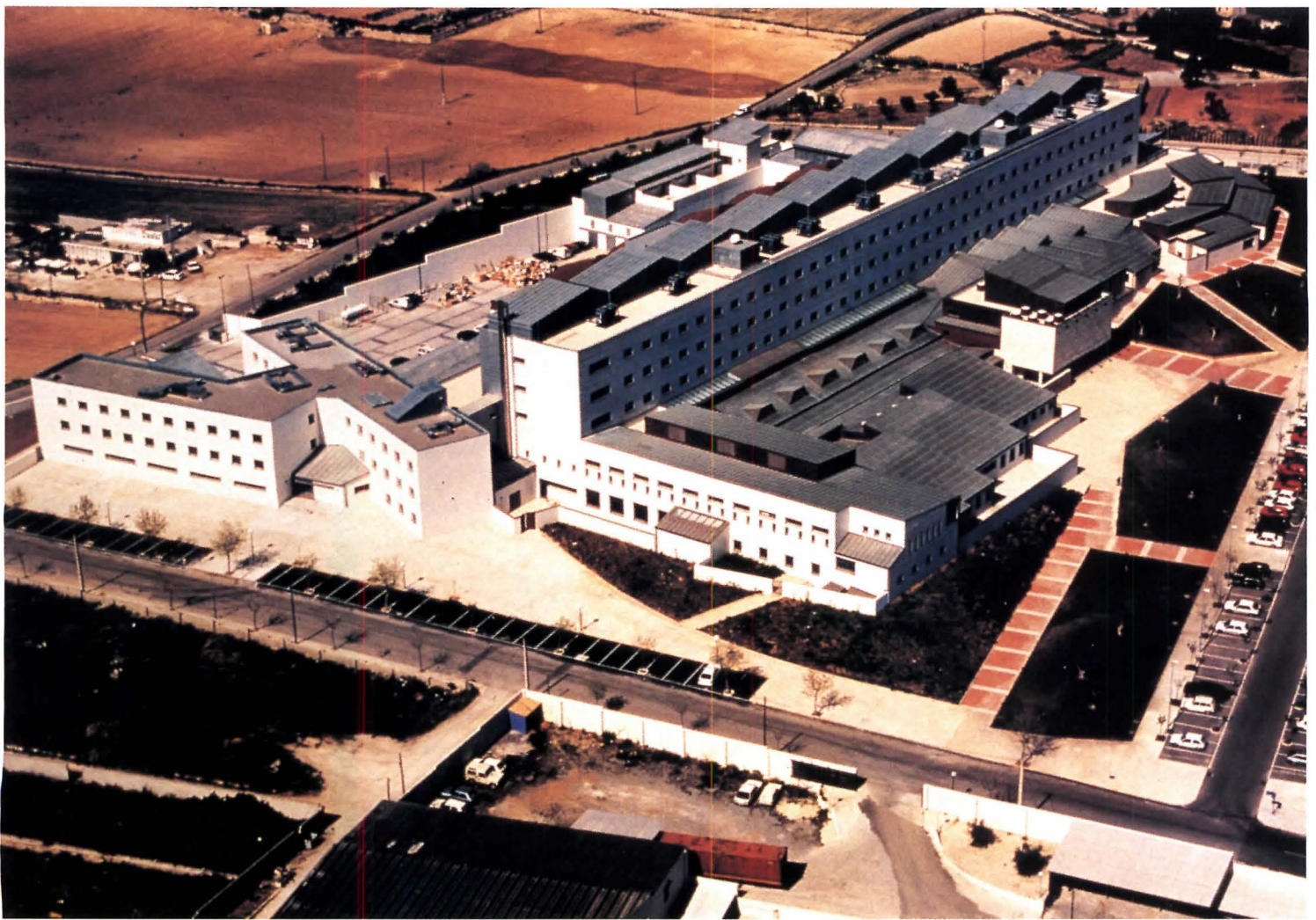
A varied expression enlivens the hospital's roofscape, from the main ward's zinc sawtooth to the copper dormers and zinc slopes over the radiology and public areas.
