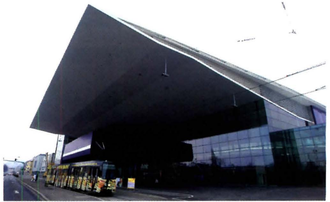
Despite a roof that cantilevers 130 feet over the street, the new Stadthalle designed by Klaus Kada maintains a human scale.
