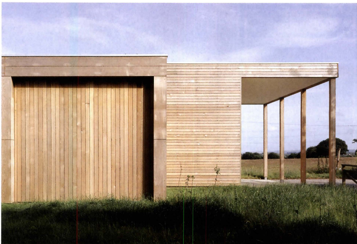
A sun porch at Faith house is defined by a setback, while volumes are differentiated by the orientation of the cedar siding.
