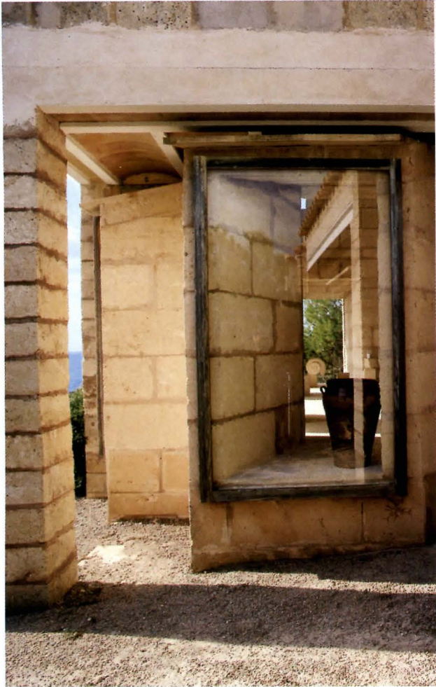
Can Lis, named for Utzon's wife, sits 65 feet above the Mediterranean on Majorca (above and facing page, top and bottom). The architect's organic modernism is steeped in time-honored construction techniques and shaped by site and local materials. Ashlar sandstone, quarried in a nearby town, is the main building block. Roof and wall openings are of reinforced concrete I-beams and lintels. Arched Catalan terra-cotta tiles span the gaps between parallel beams to make roofs (page 52). Wood frames fasten glazing to exterior walls for unobstructed views from the inside out, such as from a bay in the living room to the sea (left).
