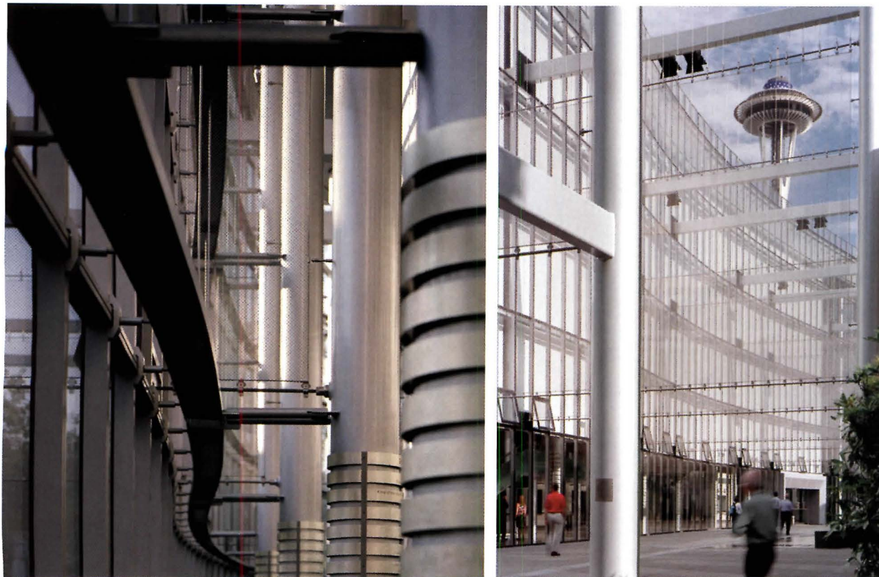
Struts and metal fittings—including a wind girt—connect scrim cables, sag rods, and a solar shade to the curtain wall and steel-clad concrete columns (left). At dusk, the scrims evolve from hues of gray to a lively ballet of color (right).
