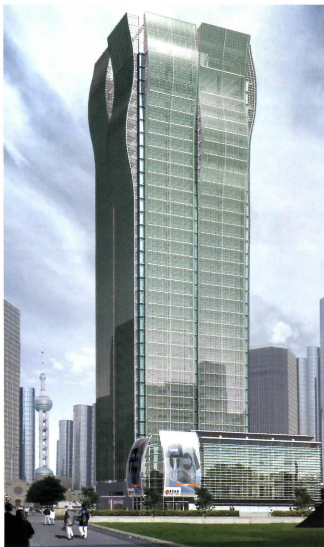
Leo A. Daly's 35-story Yinchon Cyber Tower, under construction in Shanghai, is intended to be a high-tech "intelligent building."
