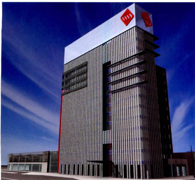
This 14-story office tower is at the center of Plaza Fundadores, a mixed-use complex under construction in northern Mexico designed by Spillis Candela DMJM.
