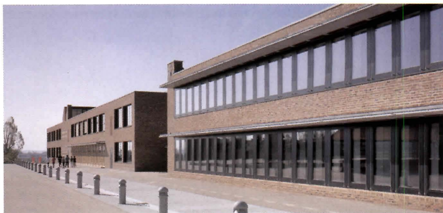
The brick courses on the face of the Scharnhauser Park Primary School (above) elegantly emphasize the horizontality of the façade design while adding texture and detail.
