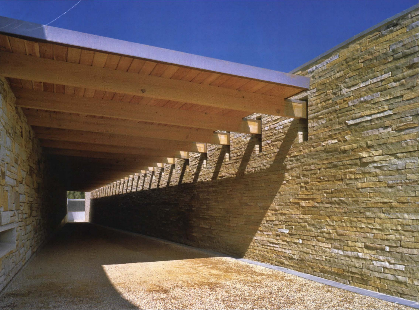
A covered passageway leads visitors from the entrance to the columbarium and a sunken courtyard.
