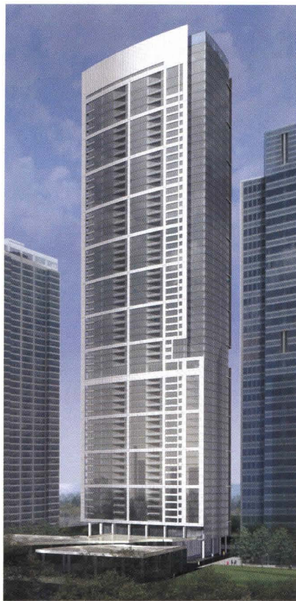
The Solomon Cordwell Buenz-designed 340 East Randolph tower in Chicago, slated for completion in 2008, underwent a battery of aerodynamics tests that affected the building's orientation, massing, and balcony configurations.
