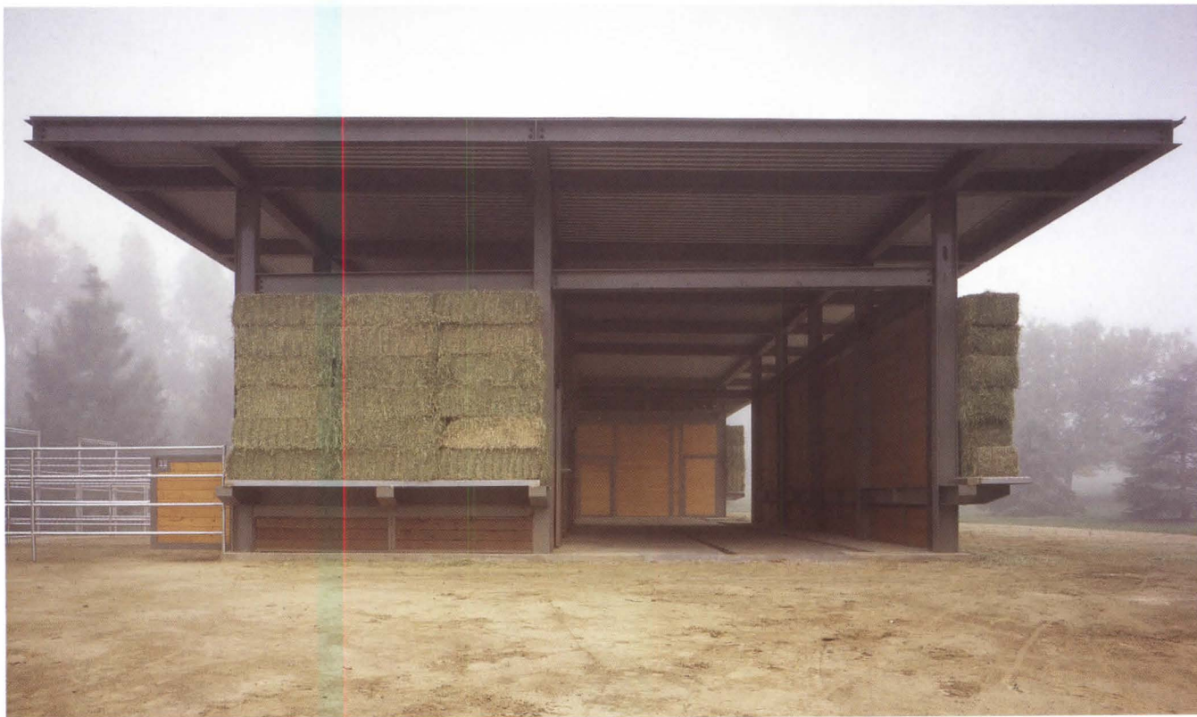
The metal roof deck extends well beyond the barn's edges to protect interior spaces and the stacked bales of hay from the rain.
