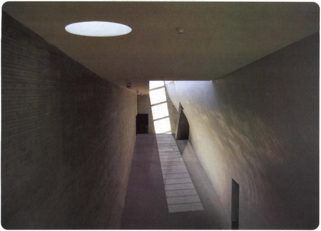
Much of the purification process takes place below ground, inside concrete boxes which are capped by a green roof; skylights emit natural light to the chambers (below).
