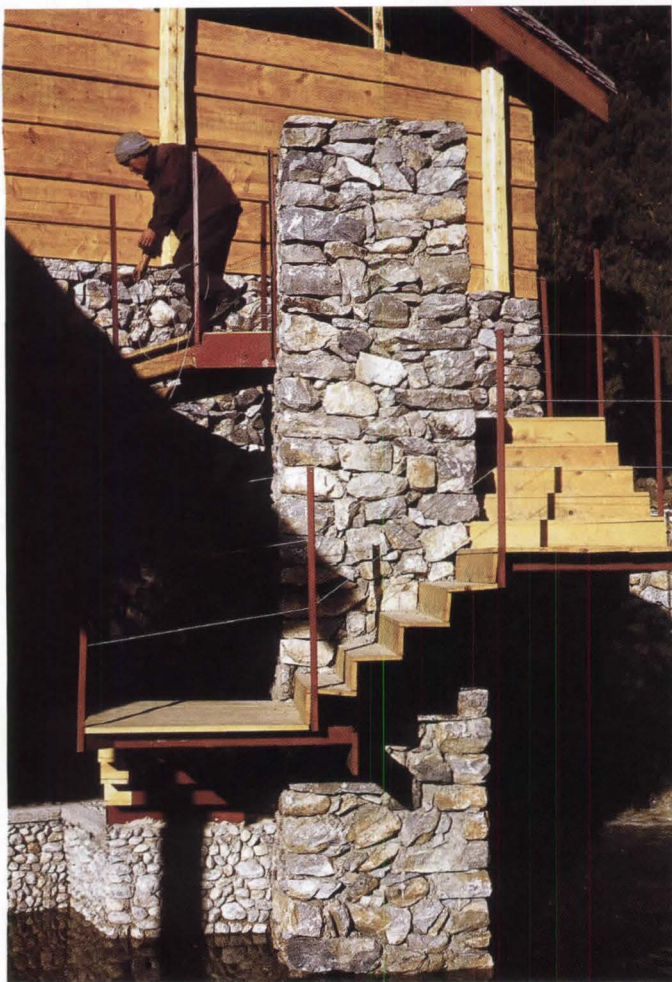
The Yuhu elementary school and community center (above and facing page) by Li Xiaodong, in the UNESCO World Heritage site of Lijiang, employs a vernacular timber-frame construction clad with nonloadbearing limestone.
