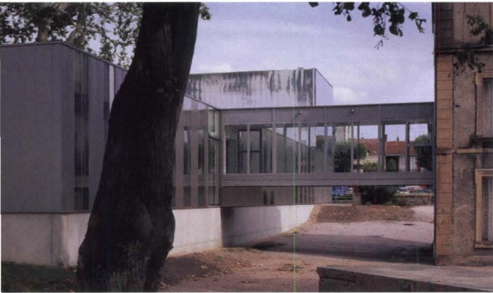
A glass-enclosed pedestrian bridge connects the new science facility to the existing neoclassical administration building (above and below left). Glass partitions are used to illuminate the interior space (bottom left), but most windows are covered with perforated steel to prevent passersby from seeing sensitive experiments (below right).
