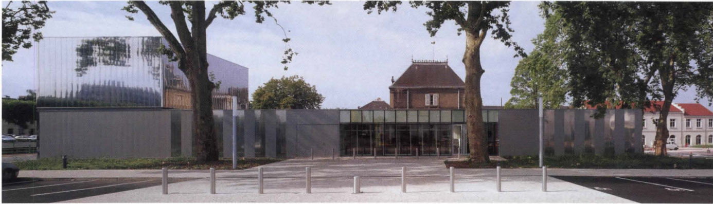
A reflective steel cladding mirrors the surrounding area (facing page) on all but the glass-enclosed entrance (above).
