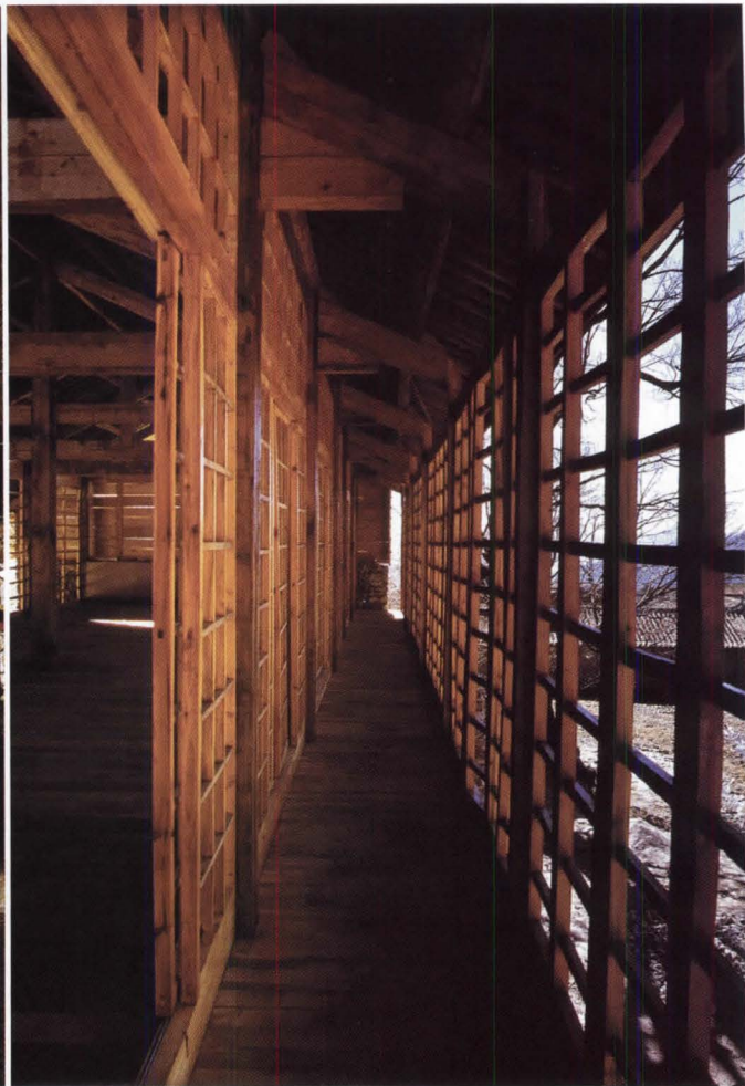
The Yuhu elementary school and community center (above and facing page) by Li Xiaodong, in the UNESCO World Heritage site of Lijiang, employs a vernacular timber-frame construction clad with nonloadbearing limestone.
