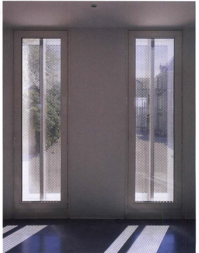
A glass-enclosed pedestrian bridge connects the new science facility to the existing neoclassical administration building (above and below left). Glass partitions are used to illuminate the interior space (bottom left), but most windows are covered with perforated steel to prevent passersby from seeing sensitive experiments (below right).
