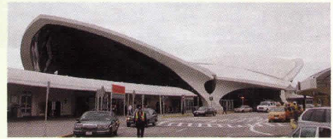
No. 115 TWA Terminal
