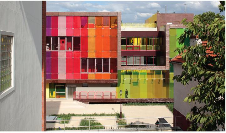
The brightly glazed Youth Center and Sports Complex in Saint-Cloud, France, is constructed from an articulated ribbon of stuctural, load-bearing, prefabricated concrete panels. This allowed for quick construction and was an experiment for Paris-based KOZ Architects, which had not previously worked with the material.
