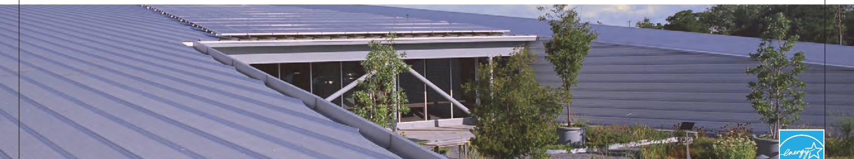
Bridges Center, Memphis, TN
