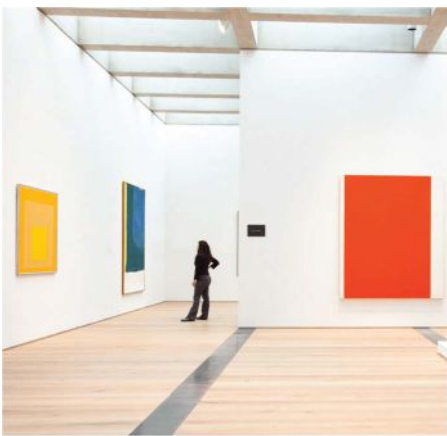
The rectilinear geometry of the concrete ceiling grid determines the position of gallery partitions and air distribution grilles in the floor.
