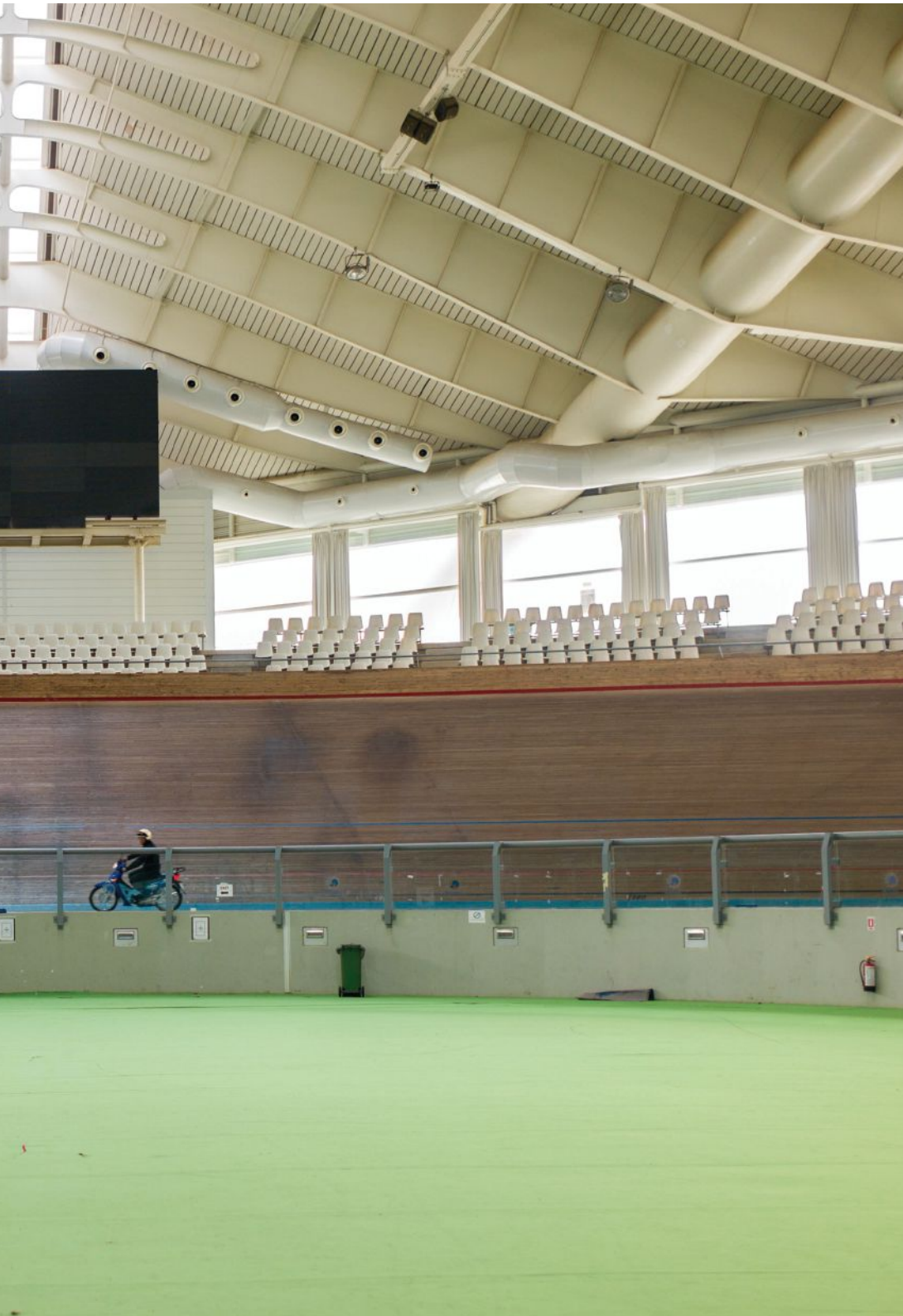
An outdoor concrete track built in 1991, this 5,200-seat facility reopened for the 2004 Games, after an extensive renovation by Santiago Calatrava, FAIA. The venue for track cycling events, it features a 250-meter banked track covered in Afzelia wood and a retractable roof supported by steel cables affixed to two swooping arches—structures that recall Calatrava's Zubizuri footbridge in Bilbao, Spain. Many facilities in the Athens Olympics Sports Complex have fallen into disrepair, but the Velodrome remains in frequent use on the European track cycling circuit.
