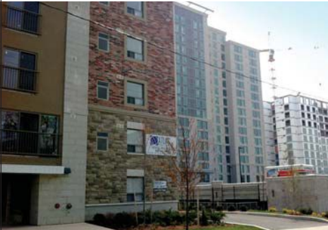
Finished and in-progress mid-rise multi-family buildings – all built with insulated concrete forms.
