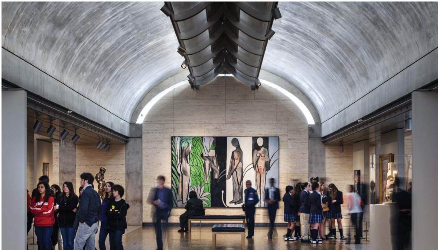
Kahn: Gallery, showing the concrete vaults and light scoop.
