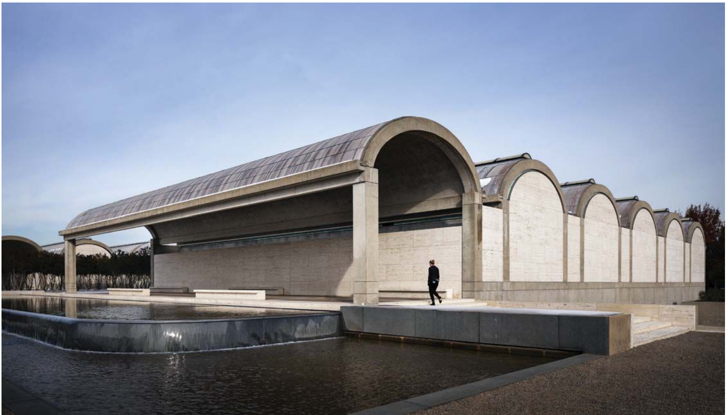
Kahn: Exterior view of the west façade and entrance, from the southwest.
