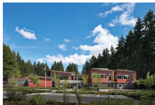
The site is so heavily wooded that it is difficult to see the building from off-site. Photo Credit: Benjamin Benschneider/OTTO
