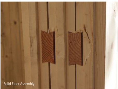
Triple-Layer Interlocking CLT Wall with Dove Tail Connection
